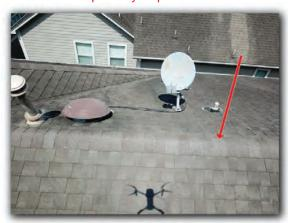
The hip and ridge shingles have reached the end of their serviceable life's as evident by excessive loss of aggregate and damage at many locations. This commonly occurs when these shingles are a different quality than the main body. Recommend contacting a qualified tradesman to evaluate the roof and make the necessary repairs.
