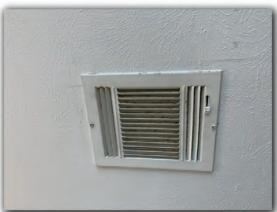
A supply register/duct was not found in the first floor study. Repair/improvement is recommended to ensure proper airflow.
