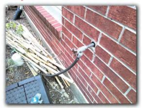
Leaks were found at the hose bib valve stems during operation of the faucets.
