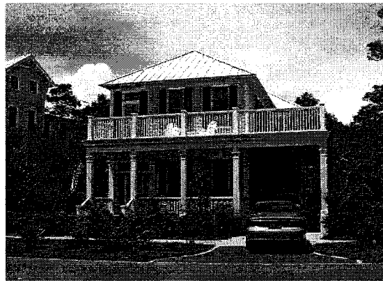
White trim, vinyl siding
