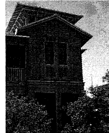
Exposed rafters are encouraged
