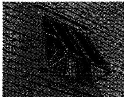
Awning shutter with simple trim
