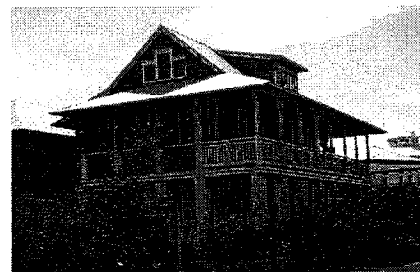
Traditional broken back roof
