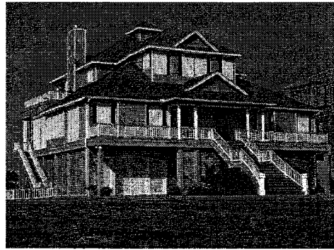
Well defined entry and use of secondary roof forms
