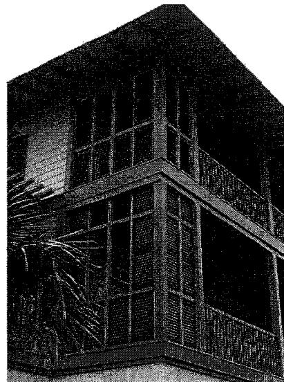
Painted porch, screens, railing and trim
