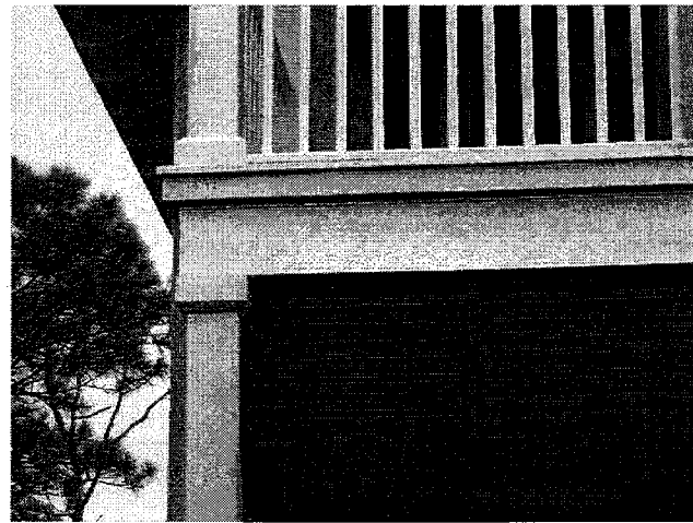
Louvered apron recessed from main body
