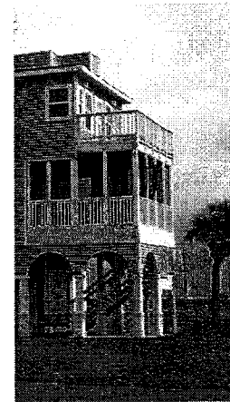
Porch integrated with structure
