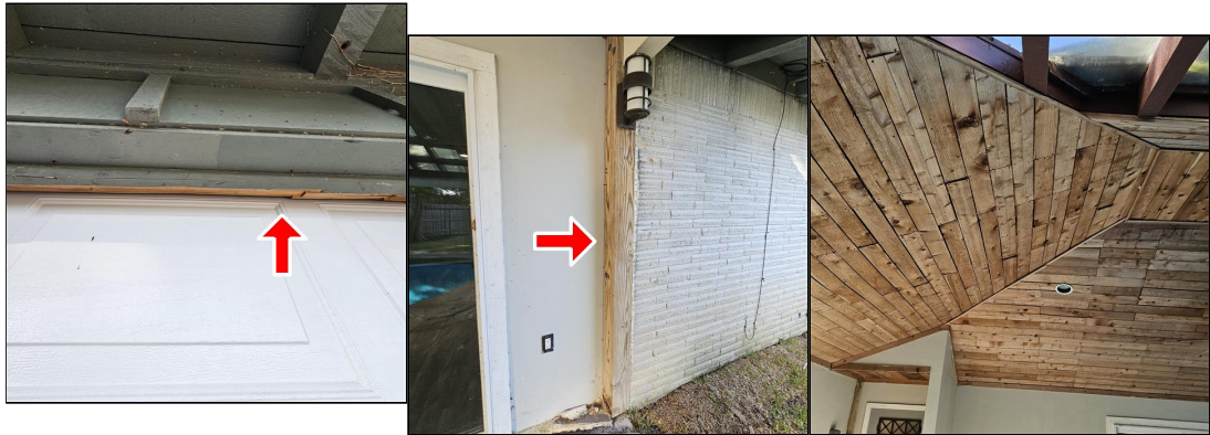
Top of garage door frame.
