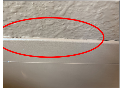
Access panel sealed
