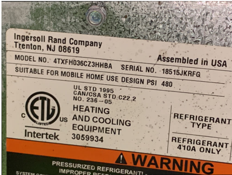
Evaporator unit 2 model and serial numbers
