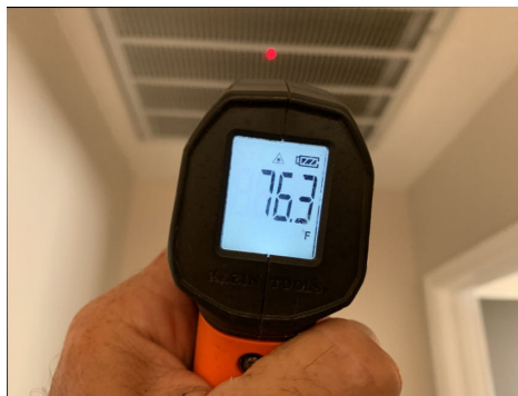
2nd floor: Return temperature
