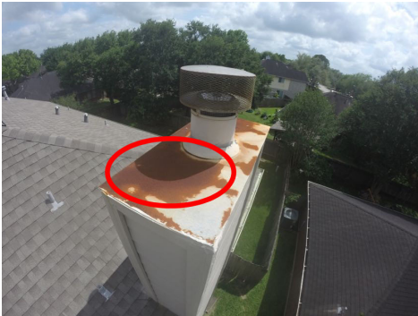
Crown deteriorated
