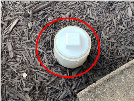
FYI: Main Cleanout located on the rear
