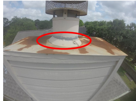
Deteriorated sealant
