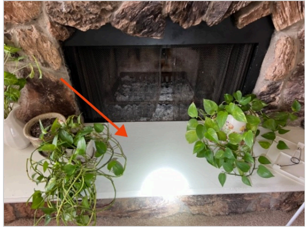
Wooden (combustible) hearth extension
