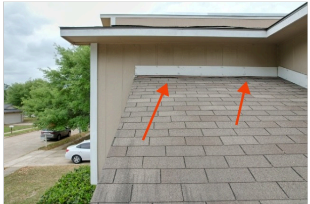
Raised flashing
