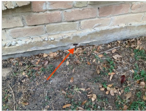
Exposed rebar
