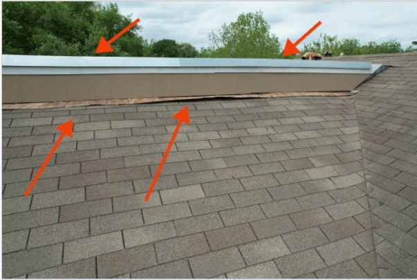
Raised flashing
