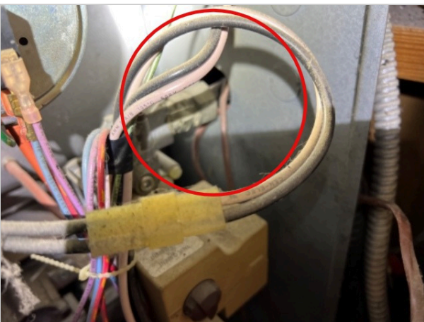
Flex line through housing
