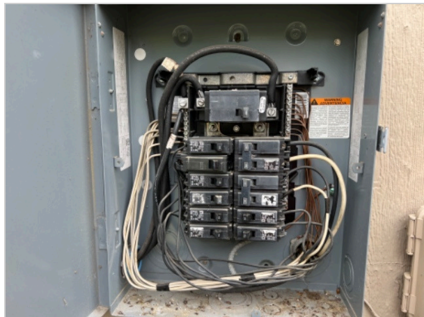
Main panel cover removed for inspection
