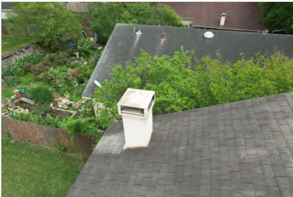
Chimney - right side
