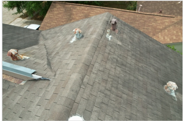
Penetrations - left side
