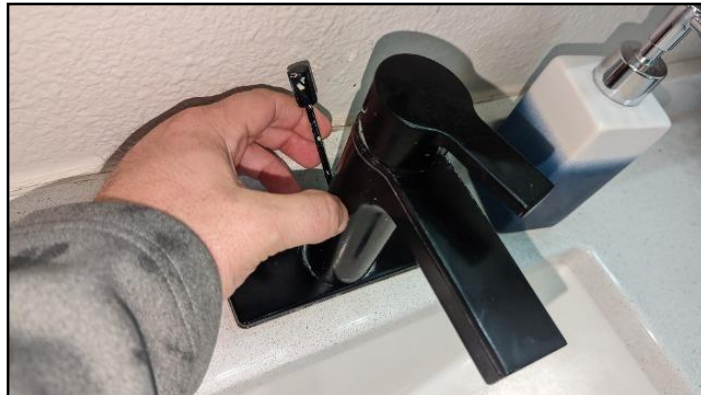
80. Drain stop ineffective
