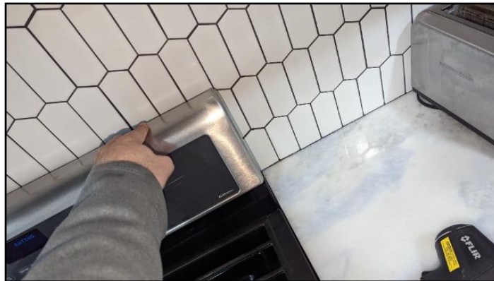
103. Anti-tipping device missing
