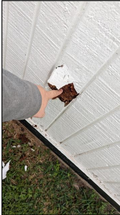
11. Rot or insect damage
