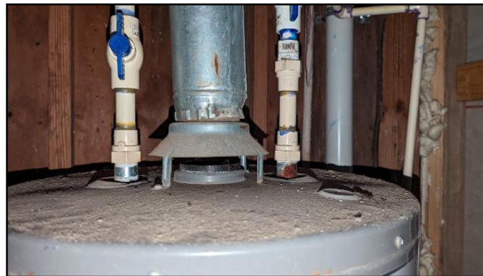
74. PVC against inlets
