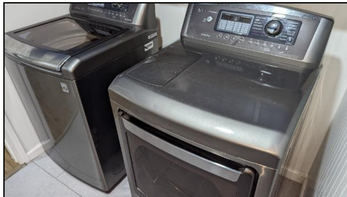
105. Drip pan missing
