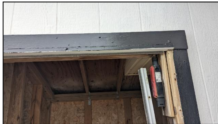
14. Rot or insect damage
