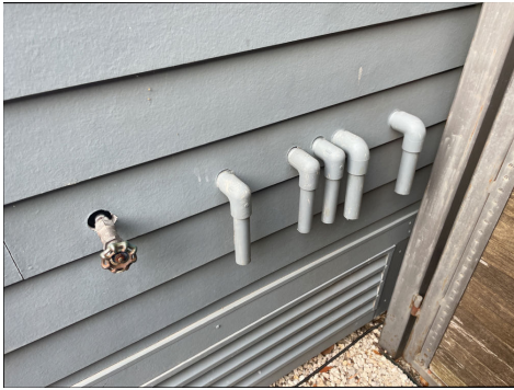
Seal exterior penetrations.
