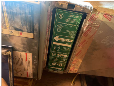
Media filters observed on all units.
