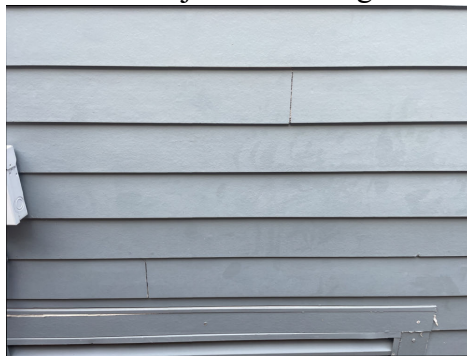
Seal joints in siding.
