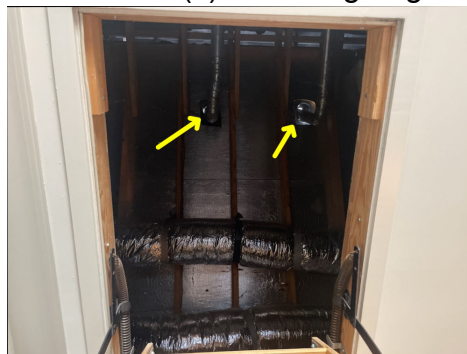
Storm collars caulked.
