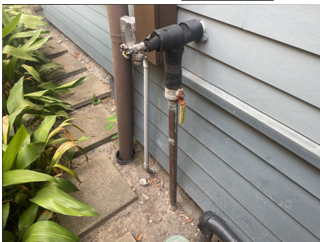
Insulate exterior pipe.
