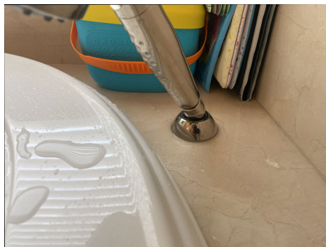
Stem washer leak at spray wand.
