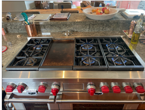
Front left burner igniter is not operational.
