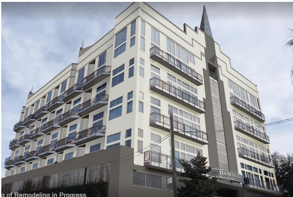
g of Remodeling in Progress
