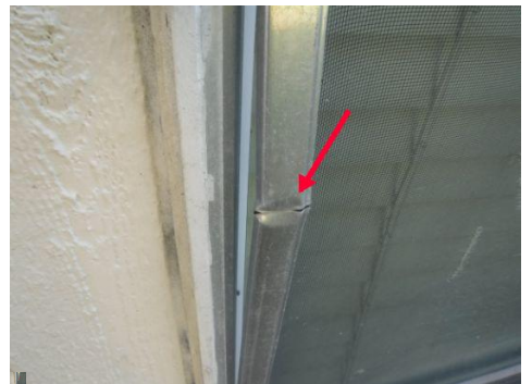
Damaged screens
