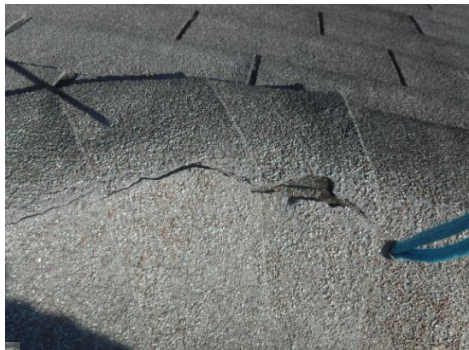
Damaged shingles
