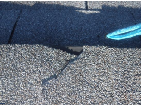
Damaged shingles
