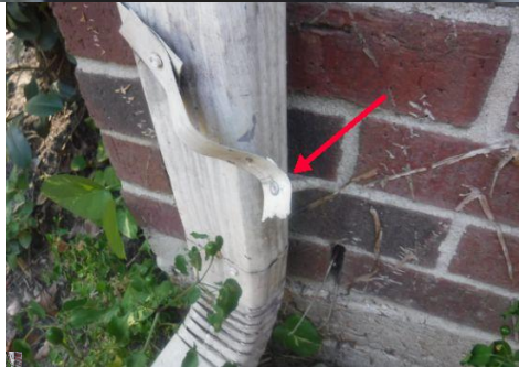
Damaged gutters
