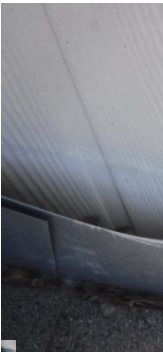
Loose flashing
