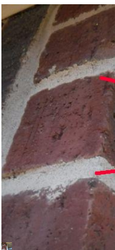
Settlement/movement crack
