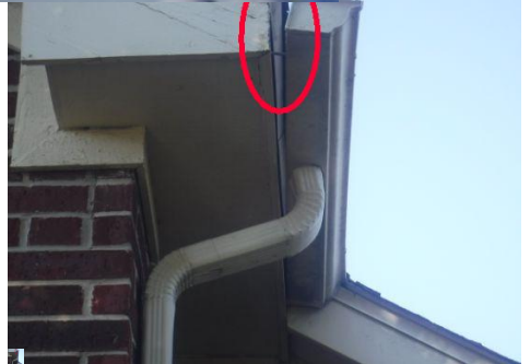
Damaged/leaning gutters
