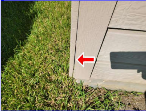
E. Item 9(Picture) Rear
