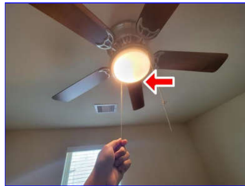
B. Item 2(Picture) Left Bedroom
