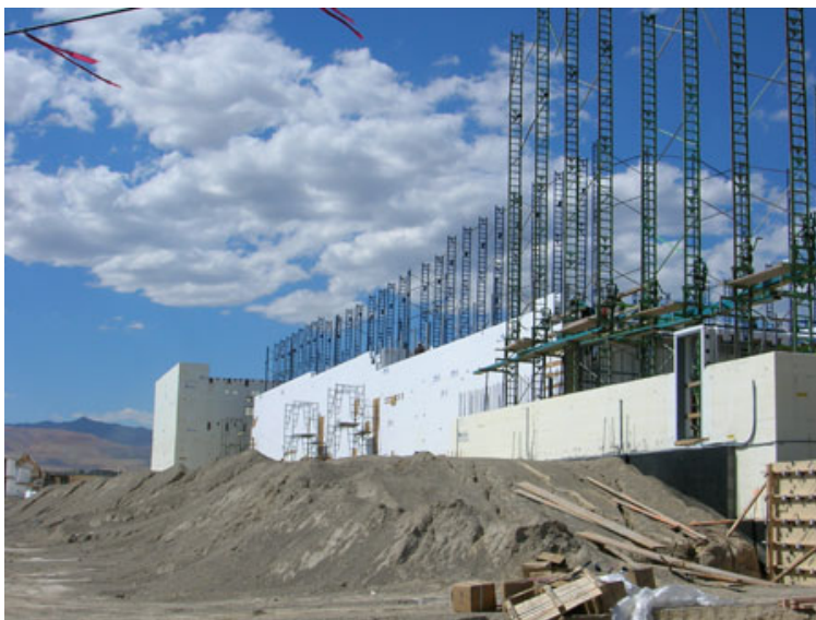
Thirty-foot tall ICF walls for multi-screen theatre project in Utah.
