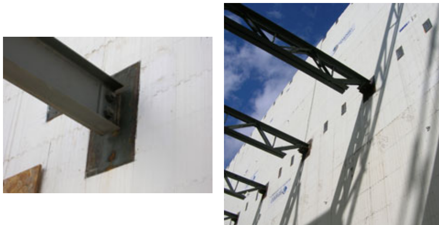
Embedded weld plates for structural steel support
