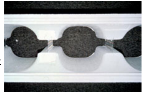
Waffle grid ICF block creates variable concrete wall thickness
