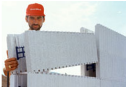
Stacking preassembled ICF formwork
