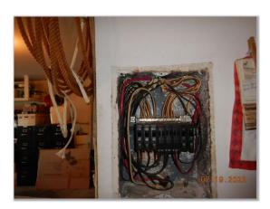
All sub-Panels require a 4 wire system, two hot wires one neutral and a ground wire. The ground wires and neutral wires have to be separated. The ground wires on the ground bus bar can have two wires in each hole, but the neutral bus bar can only have one wire in each hole. I recommend a qualified electrician correct as required. Texas Real Estate Standards of Practice now require this item to be marked as deficient.if not present
