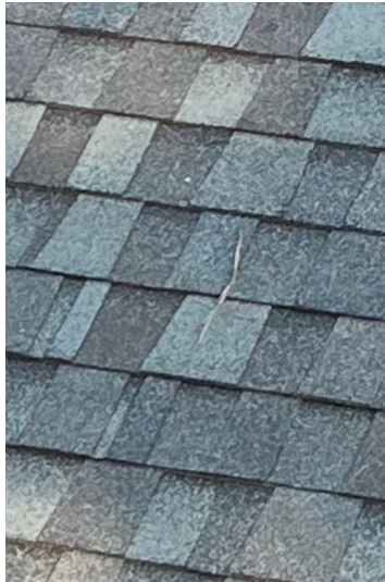
Picture of roof
