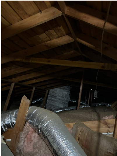
Picture of attic space
