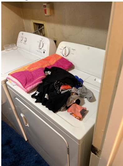
Electric and gas dryer connections present.
