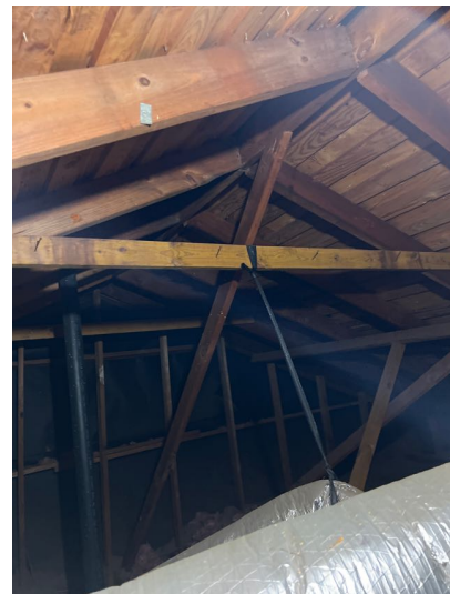
Picture of attic space
