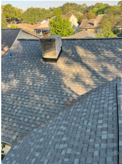
Picture of roof
