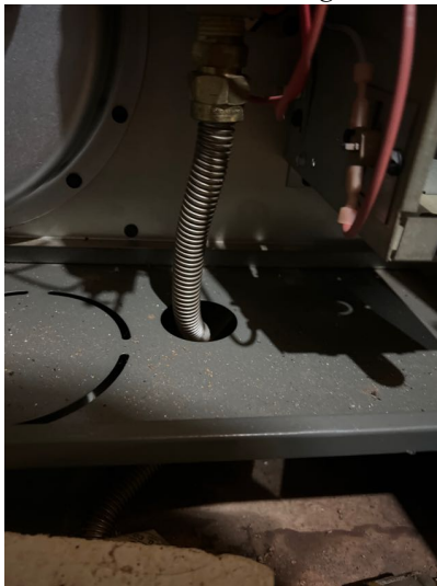
Gas connector has been installed through furnace cabinet.
