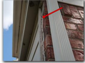
Caulking / sealant is separated or missing in some areas
