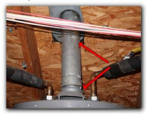
☑ Vent pipe needs adjustment and missing strap
