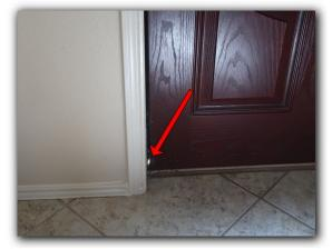
Damaged, missing weather strip at front door
