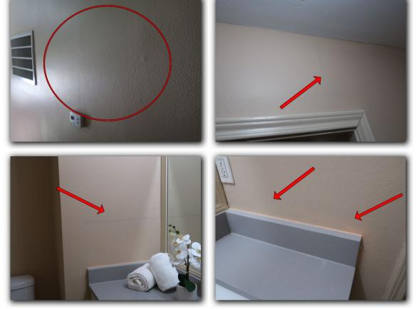
☑ Visible tape joints, patches, stains, poor finish in some areas
