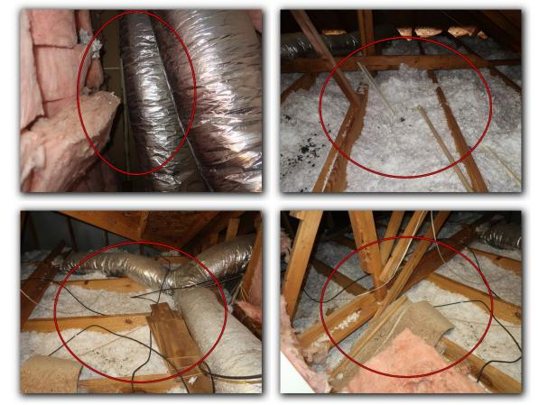
$\blacksquare$  Evidence of insulation voids and poor installation
