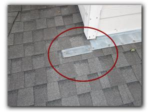
☑ Flashing is lifting, ill configured
