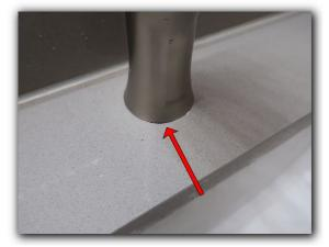
$\blacksquare$  Missing caulking and or poor installation sink faucet hall bathroom
