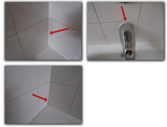
☑ Caulking or grout missing or damaged at primary bathroom
