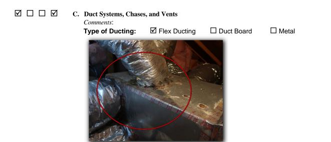
Evidence of excessive condensation / bio-growth on ducts and or plenum
