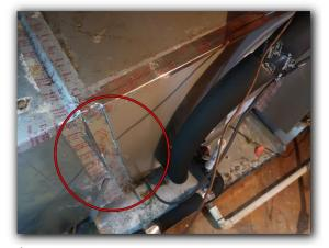
Evaporator coil is not properly sealed
