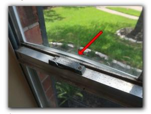
Caulking / plastic , etc. damaged and or missing
