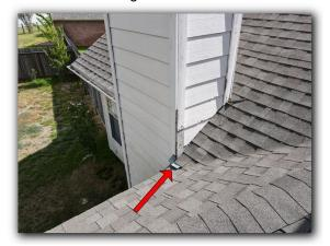
${\ensuremath{\overline{\!\!\mathcal M\!}}}$  Brick chimney not properly flashed and or lifted flashing
