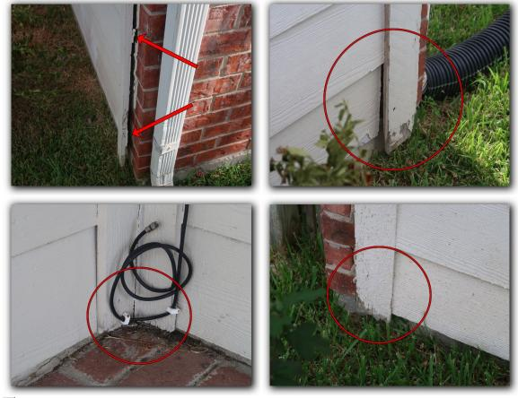
${\ensuremath{\overline{\!\!\mathcal M\!}}}$  Damaged, separated, stained, poor finish cement board siding and trim boards
