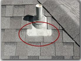
Roof penetration(s) not properly caulked / sealed
