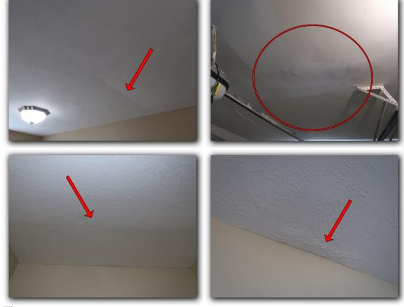
$\blacksquare$  Ceiling cracks, tape joints, nail pops, patches, stains and or poor finish in some areas
