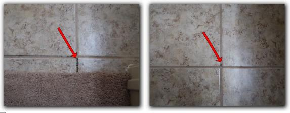
$\blacksquare$  Cracked, loose, poor installation tile and missing grout kitchen, entry and bathrooms
