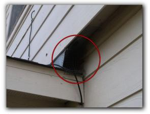
${\ensuremath{\overline{\!\!\mathcal M\!}}}$  Missing siding, trim, flashing at back patio cover
