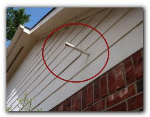
☑ Improper condensation drain line termination
