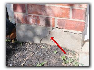
Corner cracks on foundation due to thermal expansion of bricks (cosmetic)
