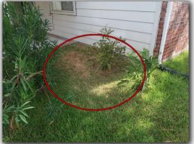
Improper drainage from foundationErosion or ponding next to foundation
