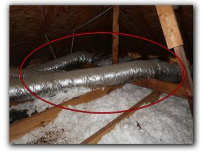
☑ Inadequate support of duct work
