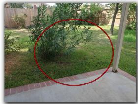
Level lot, does not facilitate proper drainage
