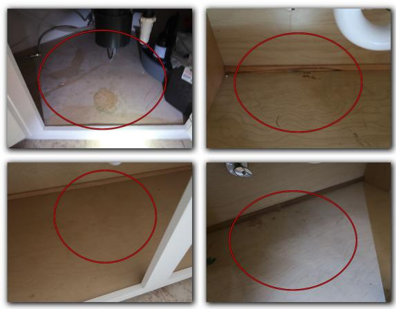
☑ Water stained, damaged, poor finish cabinet bottoms
