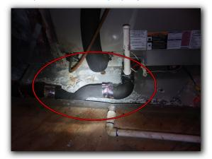
☑ Rust and corrosion in drain pan
