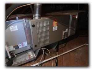
☑ Blower fan assembly is vibrating
