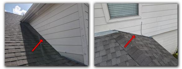
☑ Improper clearance between roof and siding
