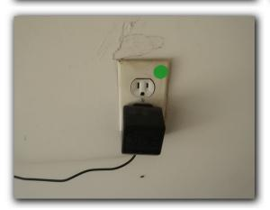
☑ No GFCI protection at one or more location. This is considered a recognized safety hazard.
