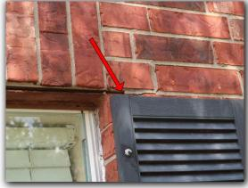
Clean and seal rusted / exposed lintels above some windows
