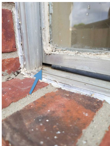
South exterior window
