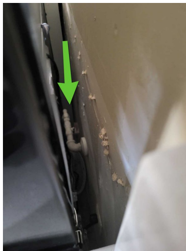
Gas shut off located behind range
