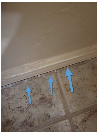
Upstairs Bathroom behind toilet
