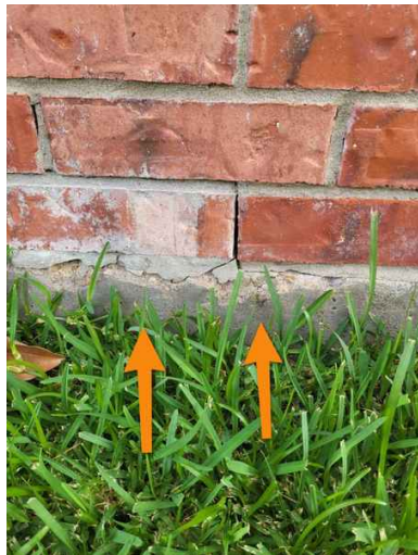
South exterior foundation
