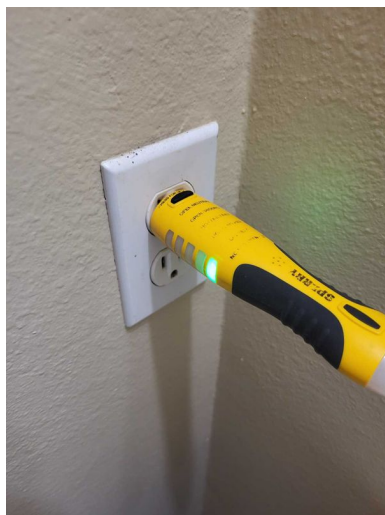
GFCI reset for half bath located in master bath
