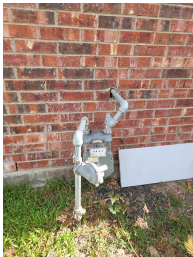
South exterior wall
