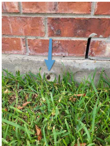
South exterior foundation
