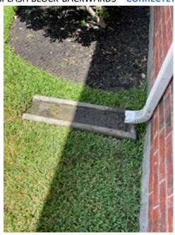
2: SPLASH BLOCK-MISSING - INSTALLED
