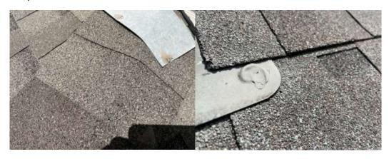
2: Rusted Roof Vent/Caps – REMOVED RUST & SPRAY COATED WITH RUST-OLEUM PAINT + PRIMER
