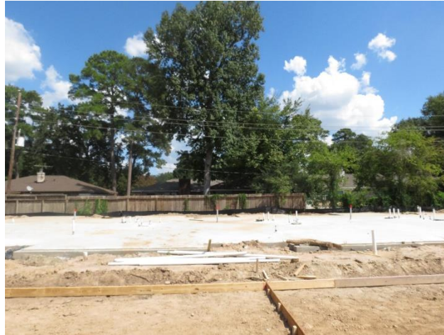
Foundations for Units 8,9 &10
