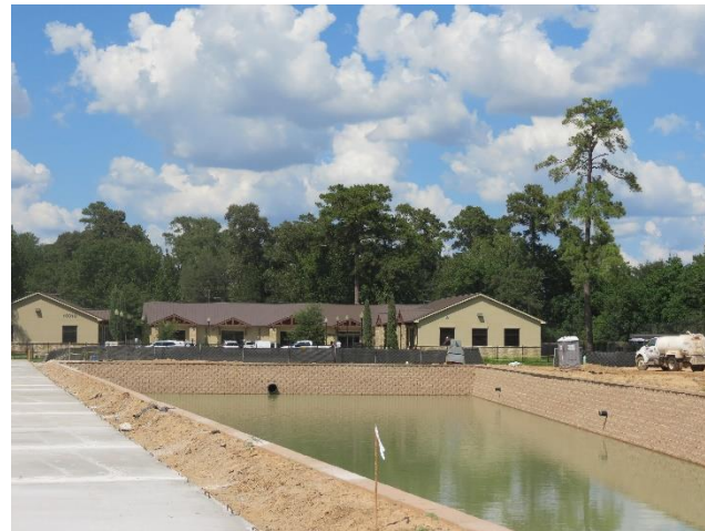
Detention Pond is Completed.
