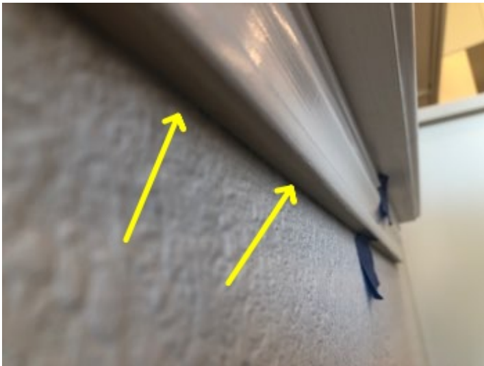
Caulk/seal underneath the windowsill apron/wall joints that are void at breakfast area, and throughout the house where needed as marked with blue tape.
