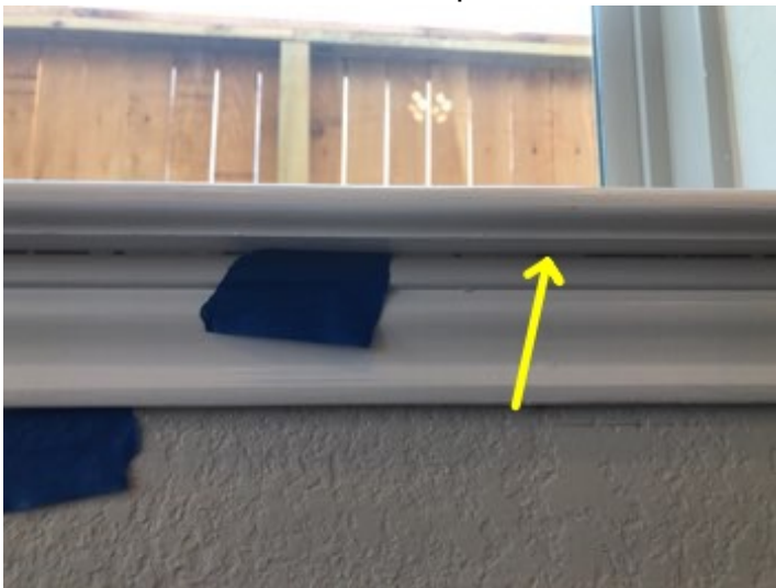
Caulk/seal below the windowsill/apron joint that is void NE of the breakfast area, and East of dining room.
