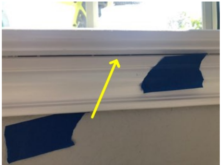
Caulk below windowsill/apron joint that is void North of dining room
