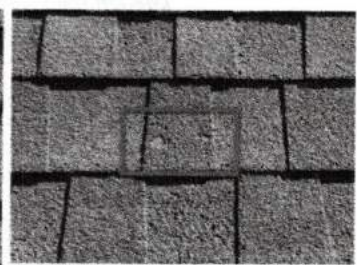
Throughout the roof of the home.
