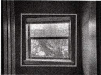
Throughout the perimeter of the home.
