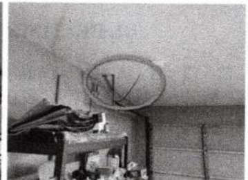
Garage ceiling of the home.
