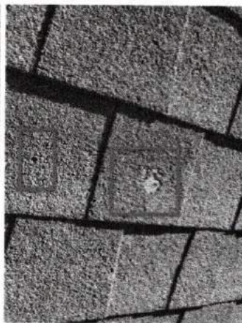
Throughout the roof of the home.
