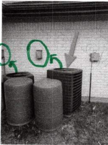
Air conditioning condenser unit needs a power cut off box.
