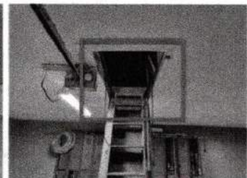
Garage Attic Access.
