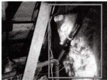
Attic above the Master Bedroom.
