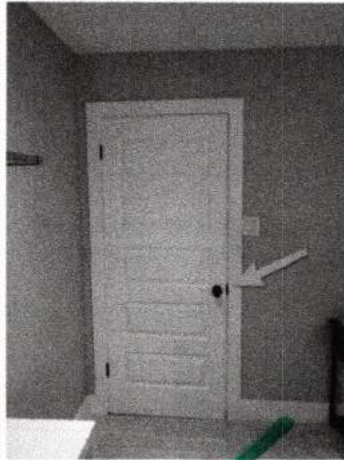
Upstairs rear left bedroom entry door.
