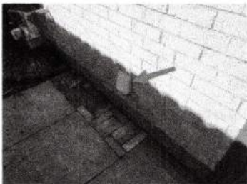
Dryer vent escutcheons on right side of the home.
