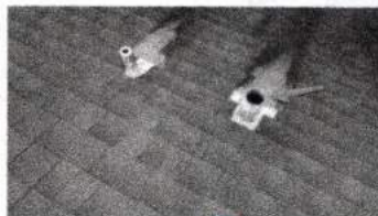
Front roof slope of the home.
