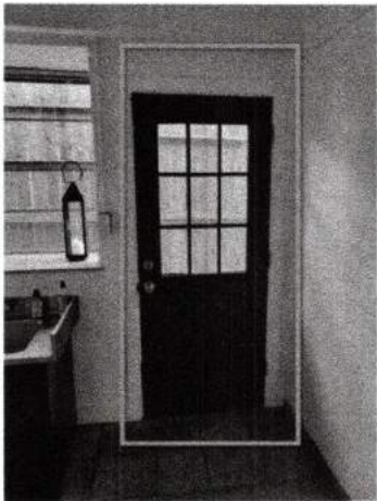
Exterior right side door.
