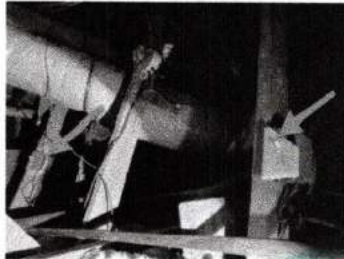
Attic above the 2nd Floor.
