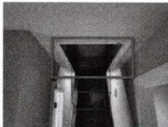
Second floor attic access.
