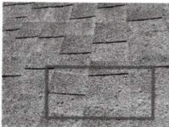
Throughout the roof of the home.
