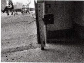
Two car garage door safety lasers.
