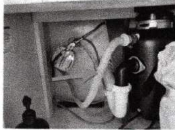
Under kitchen sink
