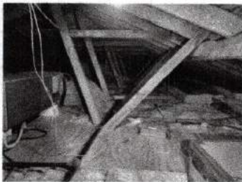
Both attics of the home.
