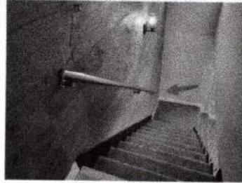
Stairway of the home.
