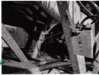
Attic above the 2nd Floor.
