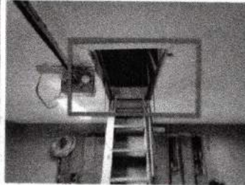
Garage Attic Access.
