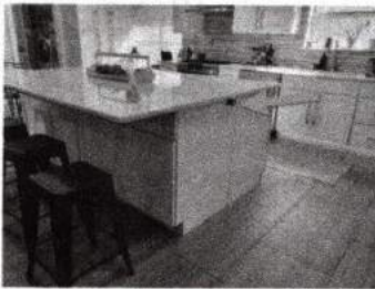
Kitchen island not Ground Fault Circuit Interrupter protected.
