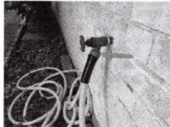
Left side of the home.
