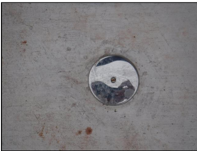
Cleanout located left front of residence.
