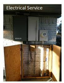
The ground wire to ground rod connection should be visible and accessible. MAIN DISCONNECT PANEL
