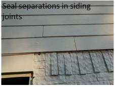
The siding manufacturer recommends a minimum siding clearance of one inch from the roofing to prevent moisture deterioration in the siding as seen in the lower edges of the siding above the breakfast room.
