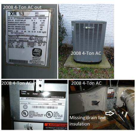
A minimum of the first ten feet of the primary condensate drain line should be insulated to prevent line sweating and dripping.
