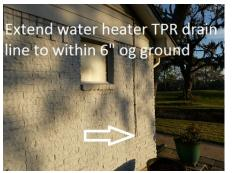
The drain line for the water heater safety pan drain should terminate within 6 inches of the ground instead of into the plumbing vent line in the attic.
