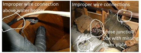
The loose upper attic junction box should be properly secured.
