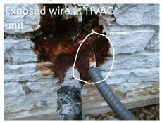
The damaged and patched thermostat wire at the outdoor unit of the central air conditioning unit should be repaired and protected from damage.
