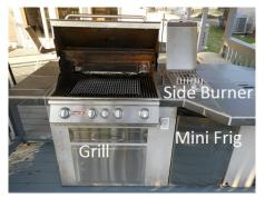
The refrigerator was unplugged and was not tested at the time of the inspection. The inoperative gas grill control knobs for the rear infrared burner and right grill burner should be repaired or replaced as necessary.
