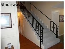
The 31 inch high stairway railings should be a minimum 34 inches high and maximum 36 inches high from the leading edge of the stairway steps.
