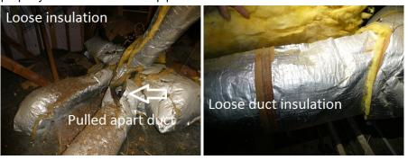
The touching and improperly suspended flexible ducts at the plenum should be suspended so the ducts do not touch. This can create a moisture/condensation issue between the two ducts. Isolation insulation should be installed between
