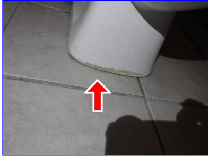
Full bathroom toilet base
