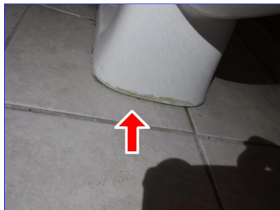
Full bathroom toilet base
