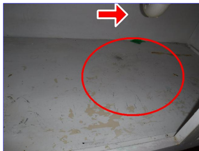
Full bathroom sink base
