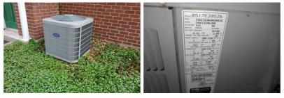
*Condensing Unit Equipment - Functional:* The condensing unit equipment was functional at the time of the inspection. The equipment responded to the corresponding thermostat, and the compressor components and fan motor components were operating.
