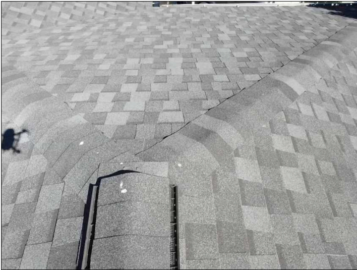
Overview of roof
