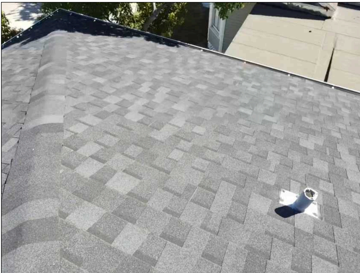
Overview of roof
