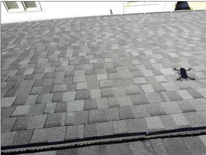
Overview of roof
