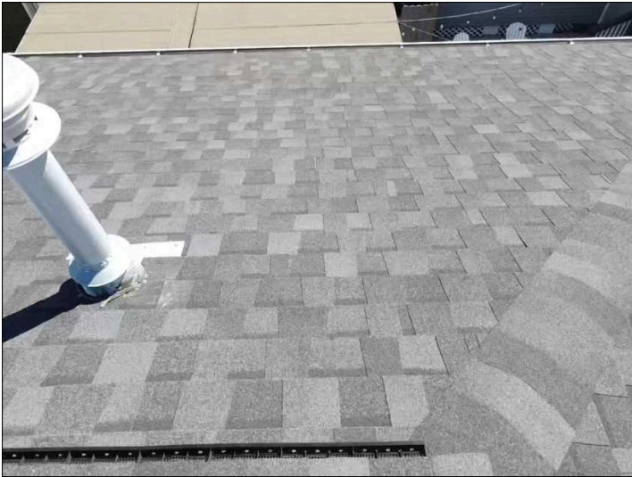
Overview of roof
