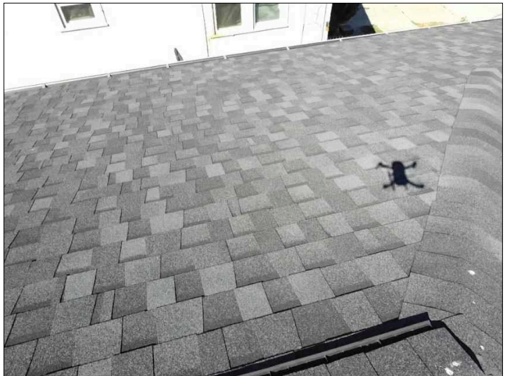
Overview of roof
