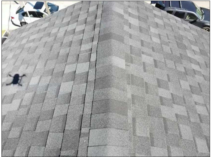
Overview of roof
