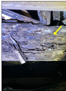
Rot/deterioration/damage beams.
