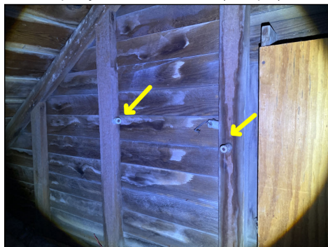
Evidence of prior knob and tube.
