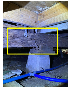
Rot/deterioration/damage beams.
