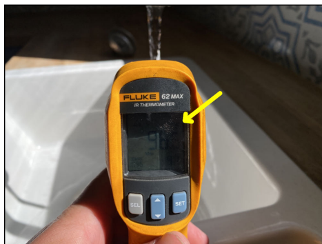
Heated water temp second floor kitchen sink.
