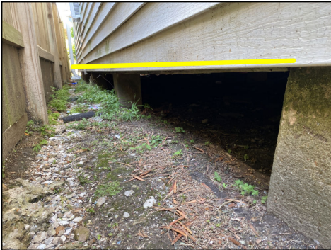
Open crawl space left side of home.
