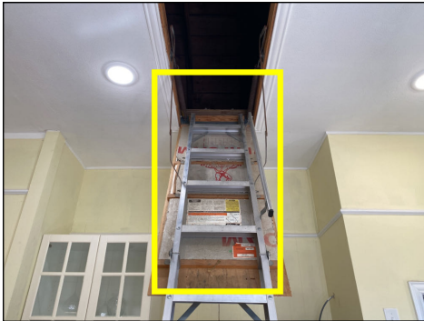
Insulate/weatherstrip attic access ladder.
