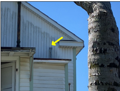
Dryer vent termination.
