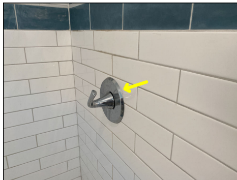
Caulk second floor bathroom shower stall.
