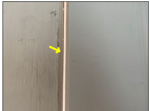
Weatherstripping front first floor door.
