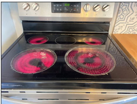
Cooktop burners first floor kitchen.
