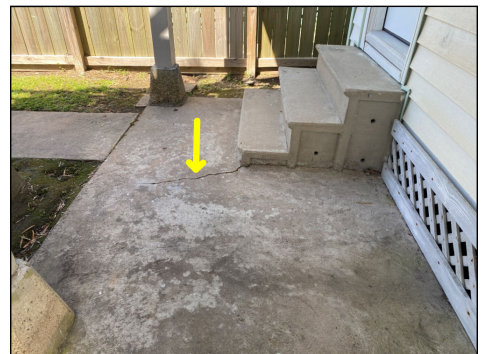
Entryway cracks.
