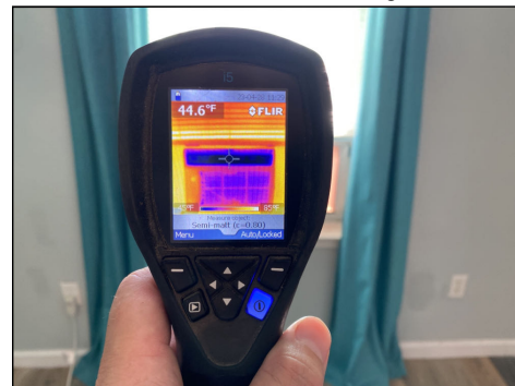
First floor front bedroom cooling.
