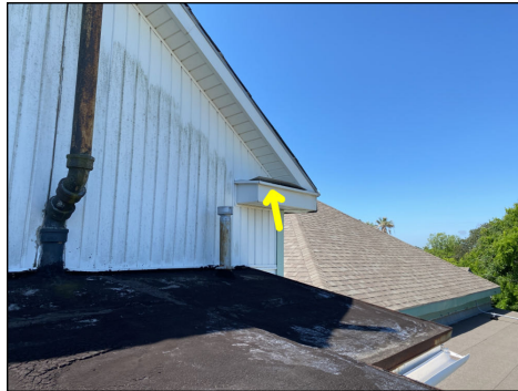
Lifted flashing.
