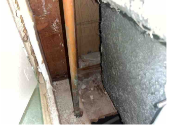
Upstairs bathroom tub drain area
