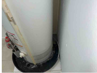
Behind water heater
