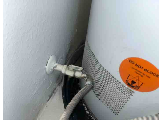
Behind water heater
