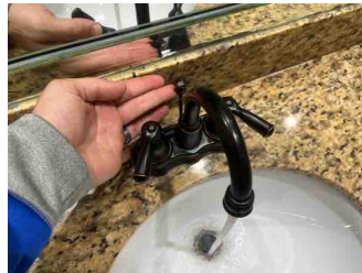
Upstairs bathroom, left sink
