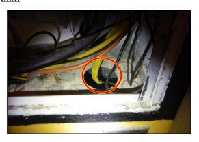
Observed two or more neutral conductors under one screw lug on the neutral bus. Current industry standards and National Electric Code permit one neutral conductor per screw lug.
