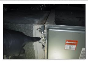
Observed metal air registers improperly install in the bathrooms. Due to excess moisture common in bathrooms i.e steam from the shower, it is recommended to use plastic registers, to prevent rusting.
