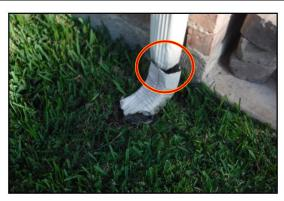
Downspouts need splash blocks at bottoms to prevent soil erosion.
