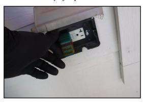
Did not observe GFCI protection of all outlets in required locations, including but not limited to the location marked below. This condition is a recognized safety hazard and needs repair.
