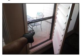
Several windows were observed to be screwed and/or locked shut. Windows in a bedroom that do not open are a recognized fire/safety hazard, including, but not limited to guest bedrooms.
