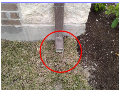
B. Item 3(Picture) left side of the home
