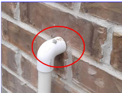
E. Item 2(Picture) left side of the home
