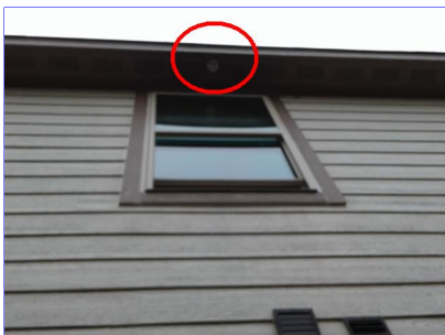
E. Item 5(Picture) left side of the home
