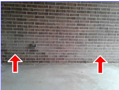
E. Item 11(Picture) multiple areas exterior
