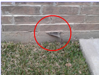
E. Item 7(Picture) left side of the home
