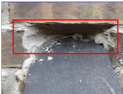
E. Item 3(Picture) left side of the home
