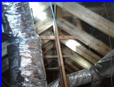
stick built with radiant barrier
