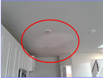
F. Item 3(Picture) kitchen
