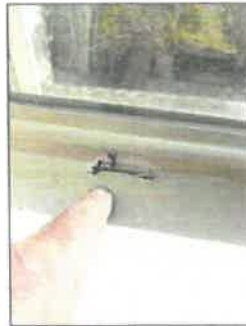
Primary bathroom, evidence of lost seal More than one window missing sensor
