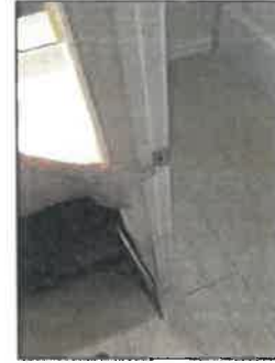
Primary bathroom, frame not plumb door binds on hinge side J&J bath, door doesn't latch needs a strike plate adjustment
