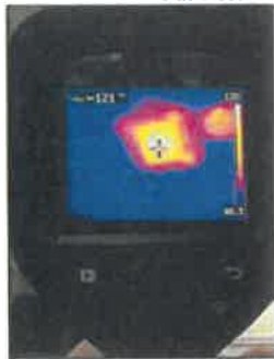
1st floor heat is functional, 121°
