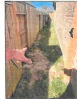
Left side, drainage via swale may need improvements
