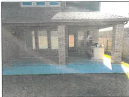
Rear covered patio and extension
