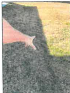
Rear, low point in swale
