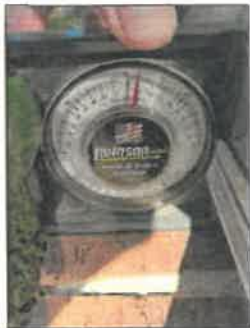
Left side, brick window sill sloped 7°
