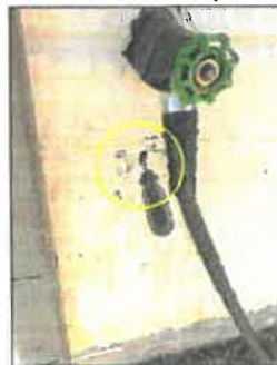
Right side, needs mortar pointing
