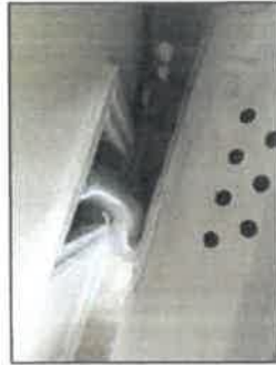
Enclosed in wall cavity and dryer installed
