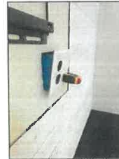
Living room, junction box not secured to stud
