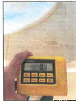
Primary bathroom W wall, -0.1
