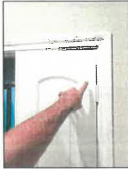
Primary bathroom, frame not plumb door binds on hinge side J&J bath, door doesn't latch needs a strike plate adjustment
