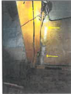
Missing insulation
