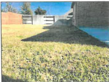
Rear, swale observed
