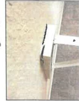
Primary closet, some of the wall mounts for the clothes hanger bar were coming loose from wall
