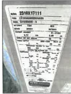
Front unit data plate: manufactured 2018, 2.5 ton, 16 seer energy rating, max 25A breaker, R-410A refrigerant
