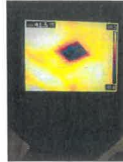
2nd floor front left bathroom, 41
