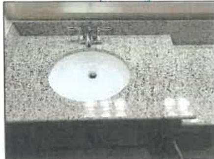
Primary bathroom, sink slow to drain
