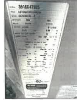
Rear unit data plate: manufactured 2018, 3 ton, 16 seer energy rating, max 30A breaker, R-410A refrigerant
