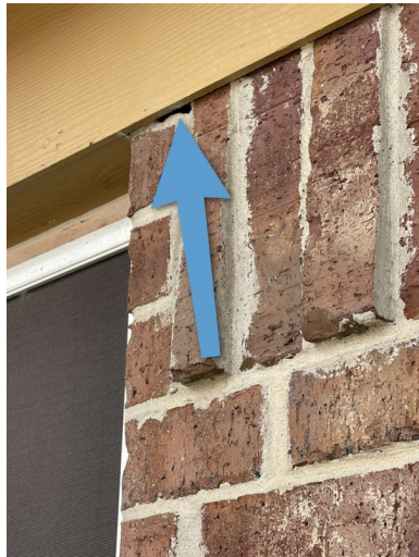
Upper Wall Left side
