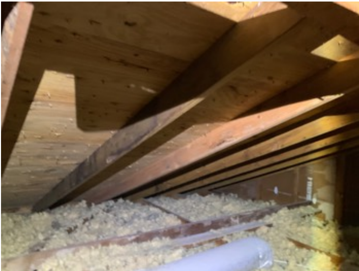
Roof Structures and Attic space
