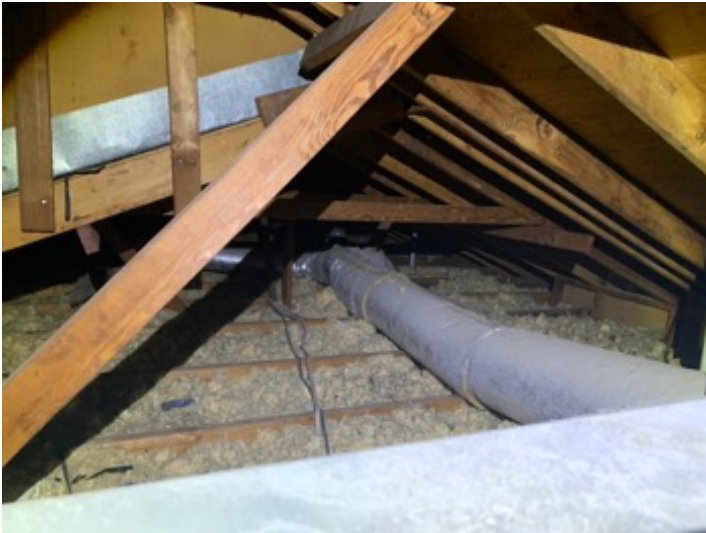
Roof Structures and Attic space
