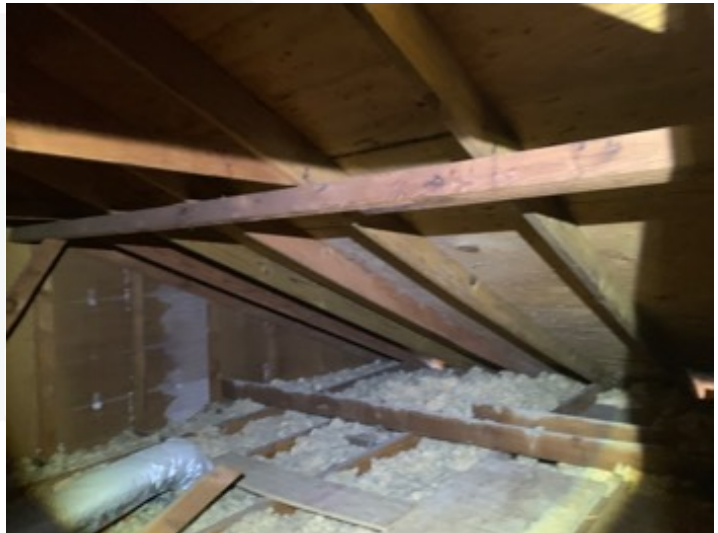
Roof Structures and Attic space
