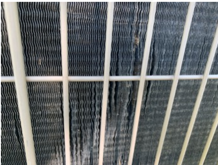
No emergency shut off switch within 50 feet of the AC unit
