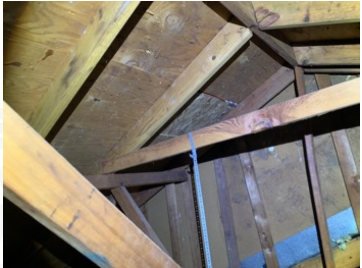
Roof Structures and Attic space
