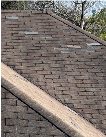
Damaged shingles.
