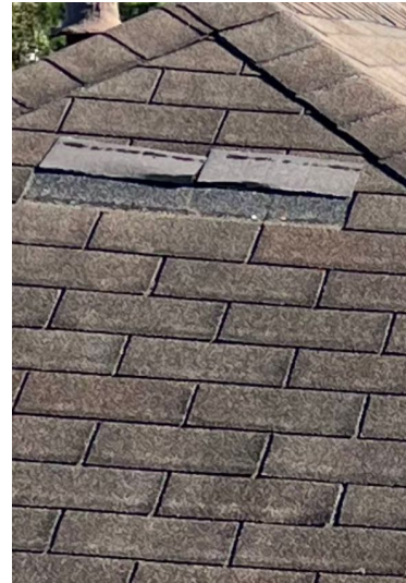
Damaged shingles.
