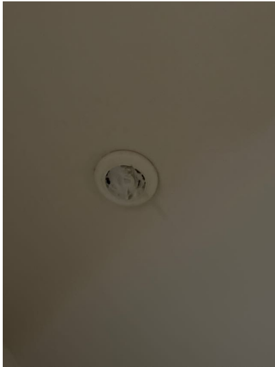
Missing smoke alarm
