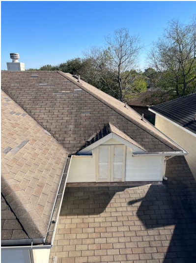
Picture of roof
