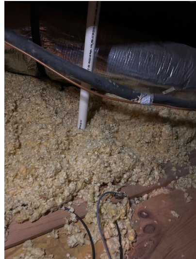
Picture of attic space
