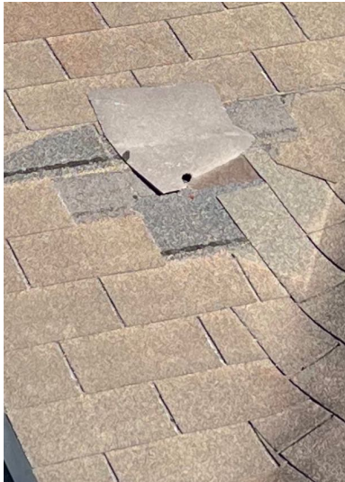
Damaged shingles.
