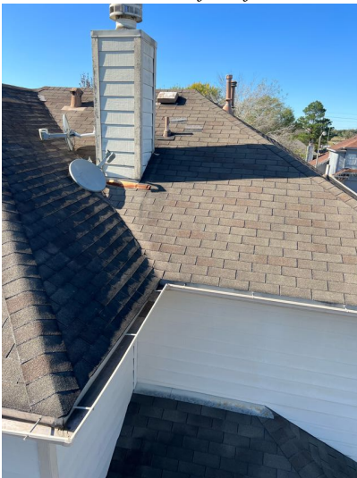
Picture of roof
