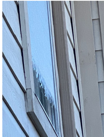
Damaged window screen
