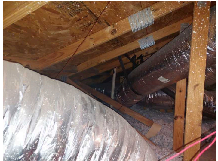
Picture of attic space
