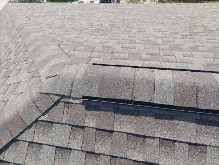
Picture of roof
