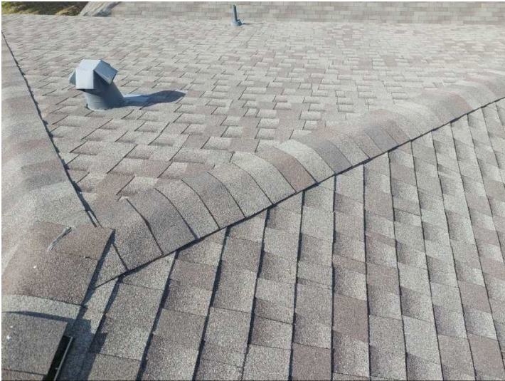
Picture of roof
