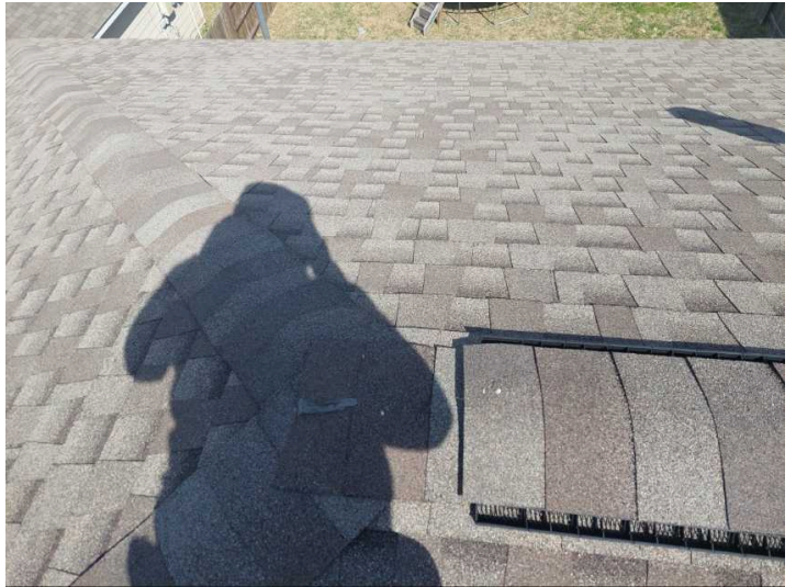
Picture of roof
