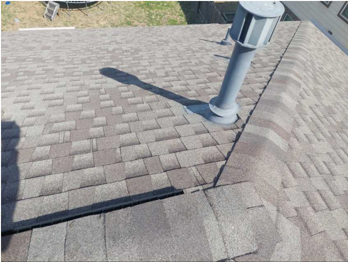
Picture of roof
