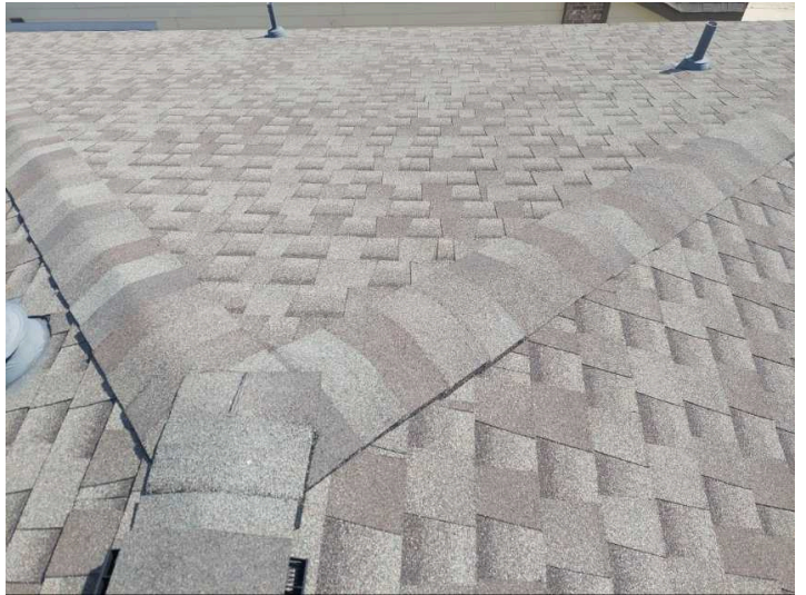
Picture of roof
