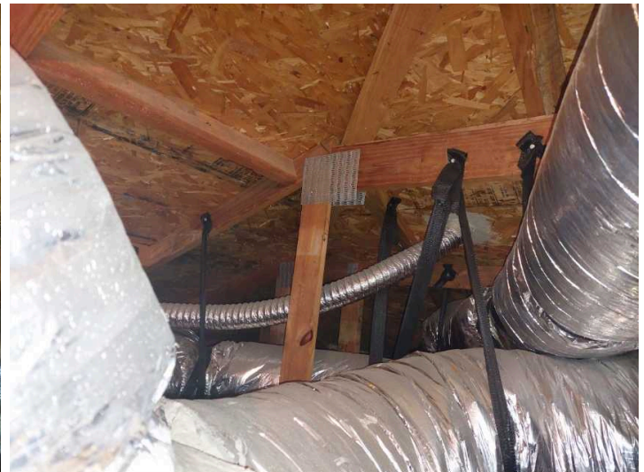
Picture of attic space
