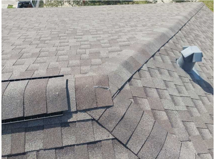
Picture of roof
