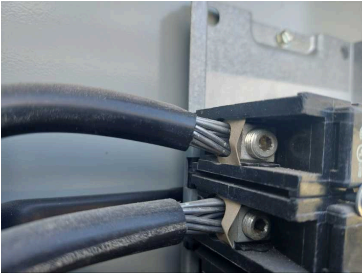
Aluminum service conductors missing anti-oxidant grease
