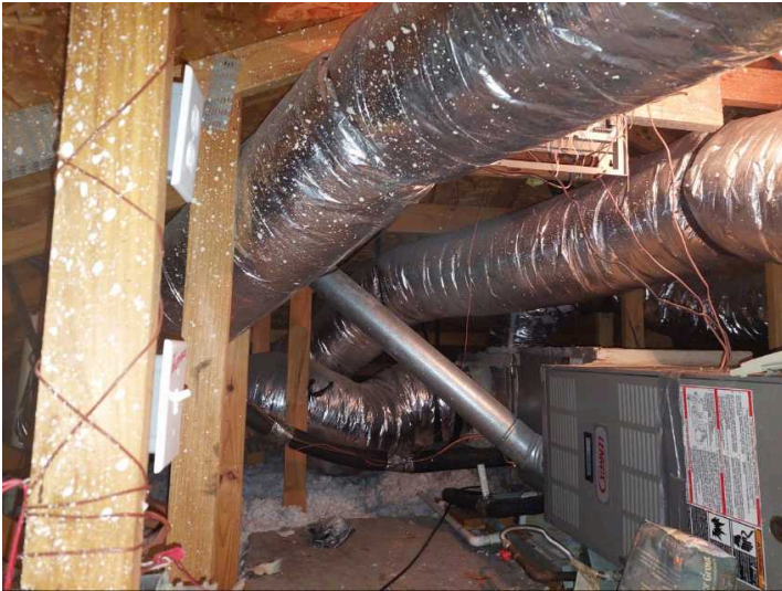
Picture of attic space
