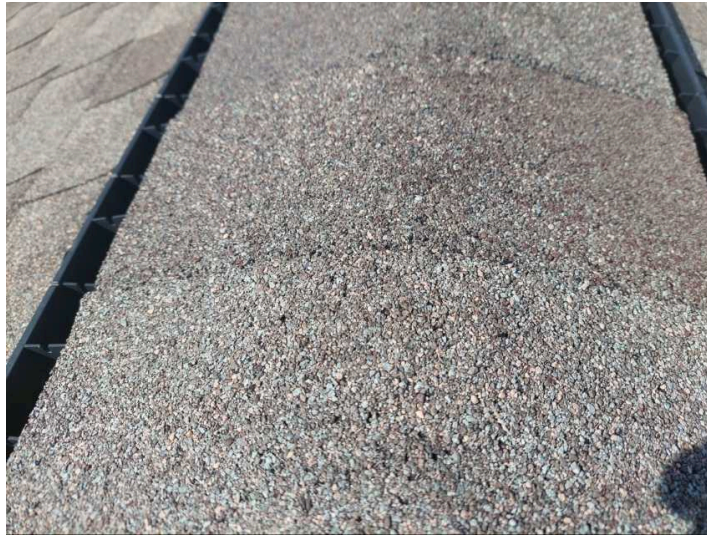
Picture of roof
