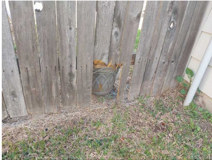
Wood pickets damaged and/or missing in fence line
