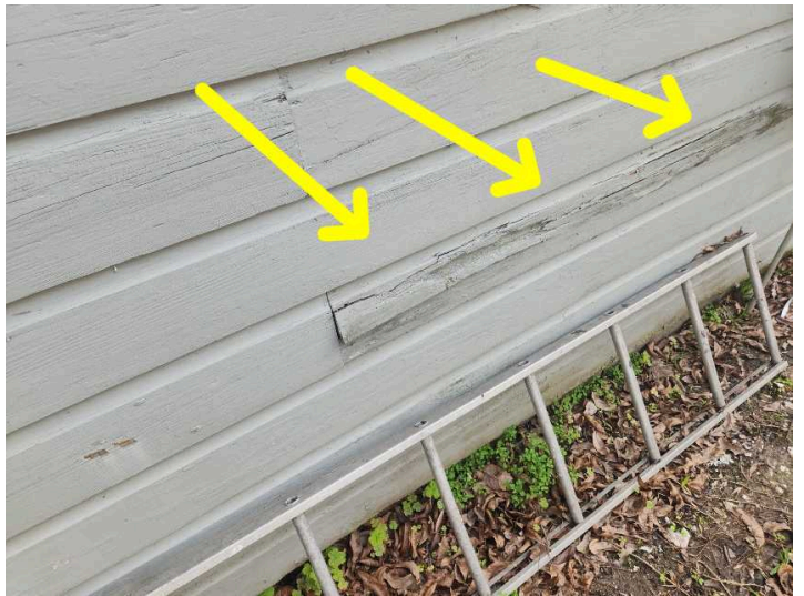
Wood deterioration
