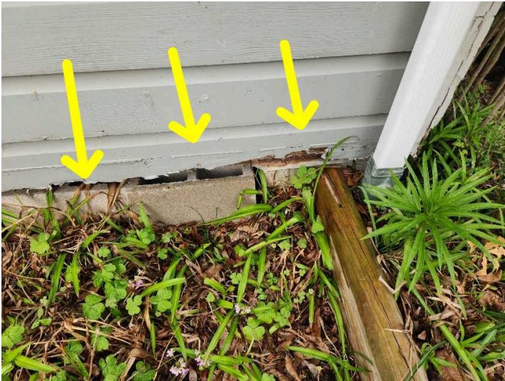
Wood deterioration
