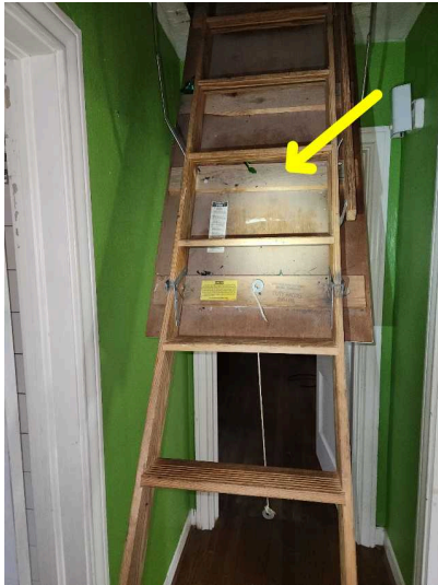
Missing insulation
