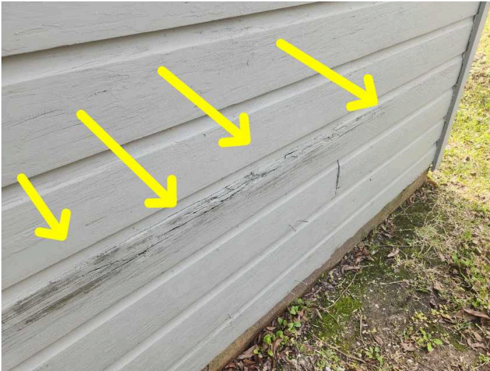
Wood deterioration
