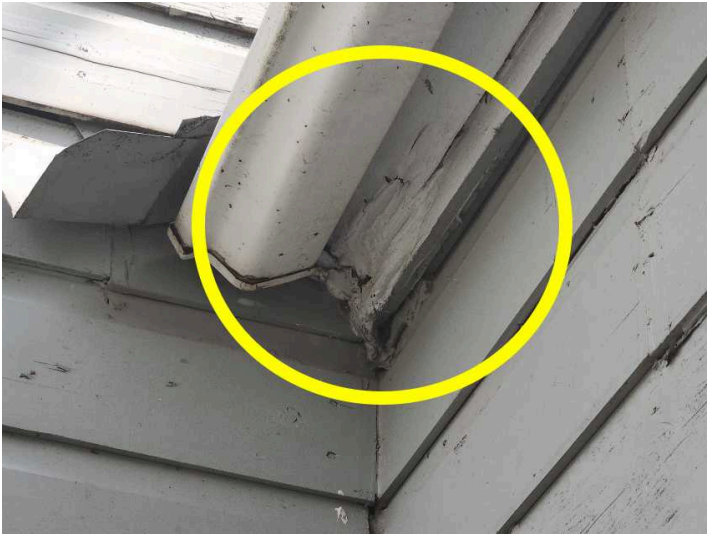
Wood deterioration
