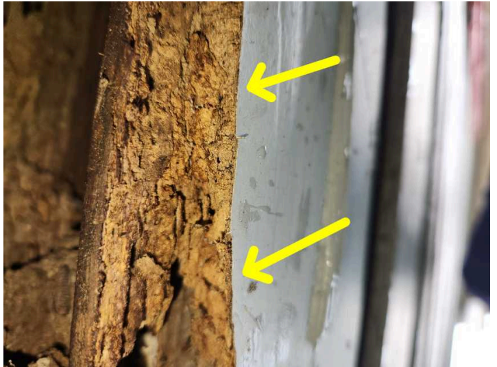
Wood deterioration
