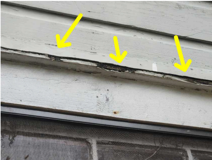
Wood deterioration
