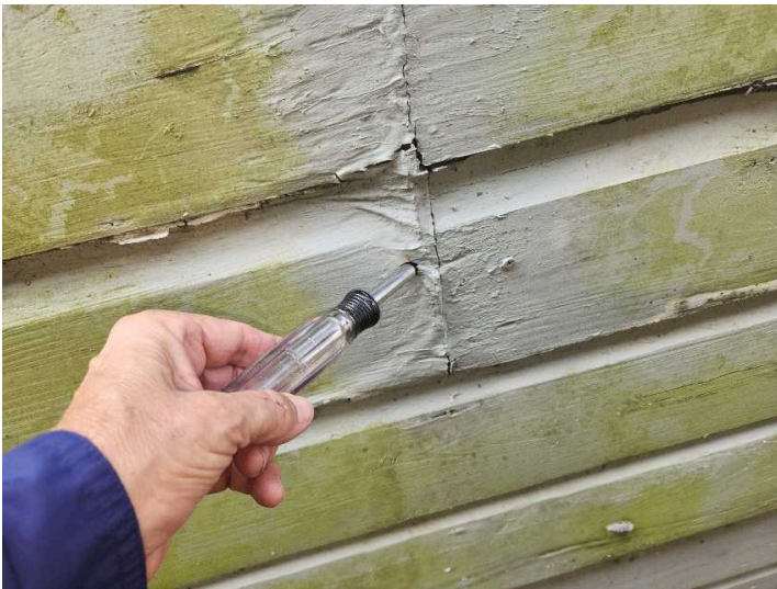
Wood deterioration
