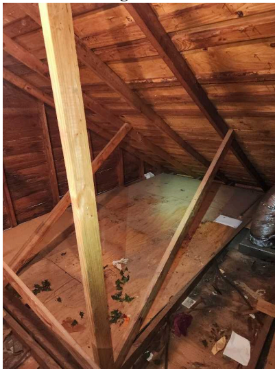
Missing insulation
