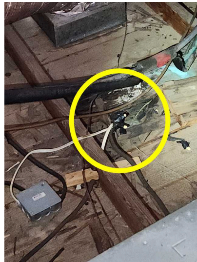
Exposed wiring
