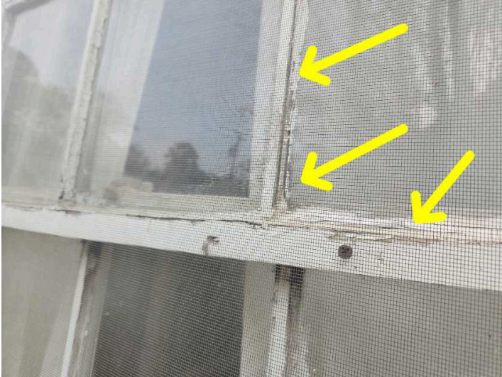
Glazing damaged
