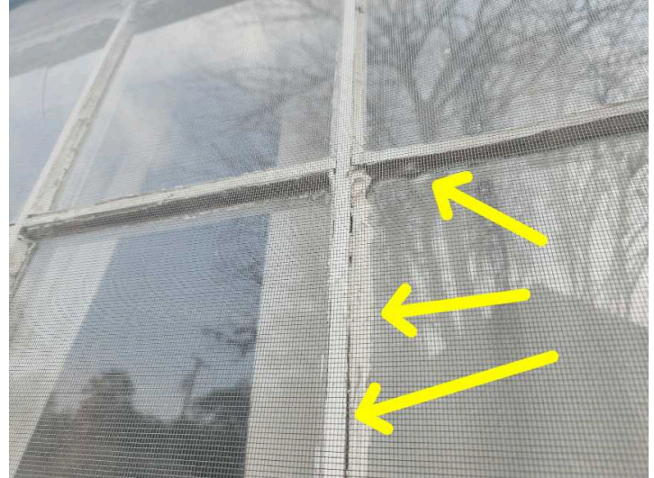
Glazing damaged
