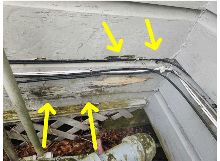
Wood deterioration
