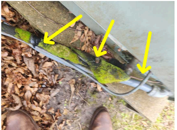
Insulation deterioration
