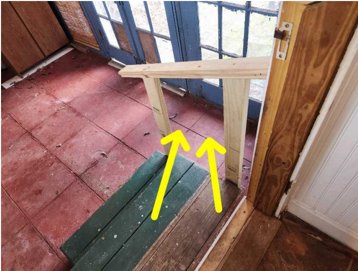
Spindles missing
