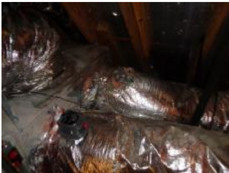
Damaged ducts
