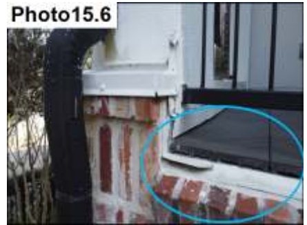
Balcony Flashing / Seal
