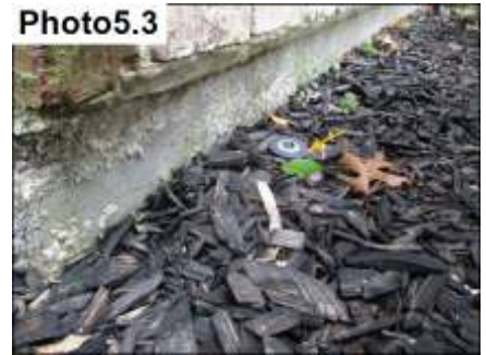
Sprinklers / Redirect as Needed
