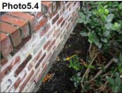
Sprinklers / Redirect as Needed
