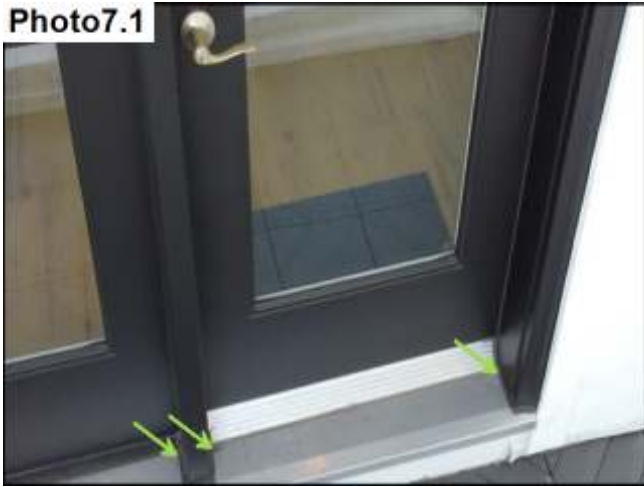
Door Trim and Miter Sealant / Maintain
