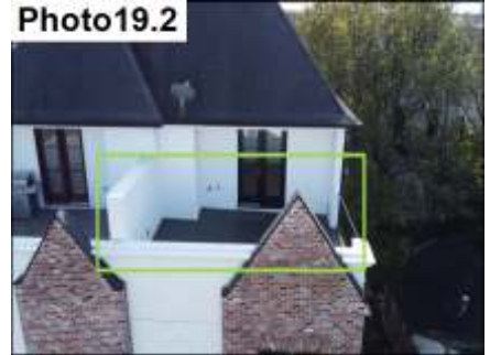
Rooftop Parapet Cap / Seal
