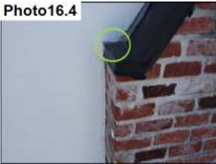
Kickout Flashing Location / Seal
