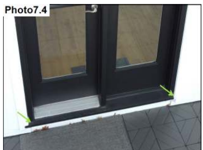
Door Trim and Miter Sealant / Maintain
