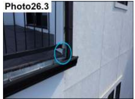
Balcony Flashing / Seal
