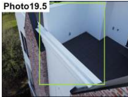
Rooftop Parapet Cap / Seal
