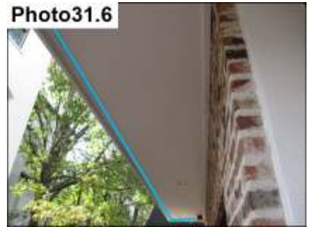
Relief Present / Clean Out Excess Sealant
