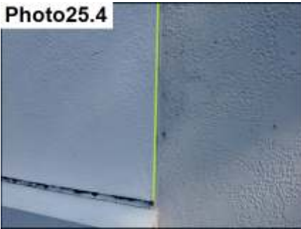
CFB/Stucco Termination / Seal
