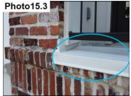
Balcony Flashing / Seal
