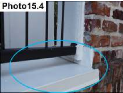
Balcony Flashing / Seal
