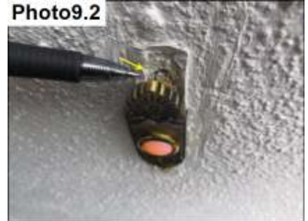
Penetration Sealants / Seal
