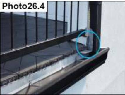
Balcony Flashing / Seal
