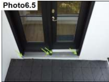
Door Trim and Miter Sealant / Maintain
