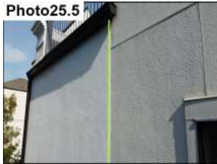
CFB/Stucco Termination / Seal
