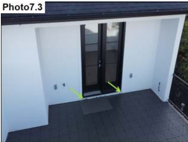
Door Trim and Miter Sealant / Maintain
