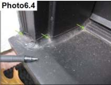
Door Trim and Miter Sealant / Maintain
