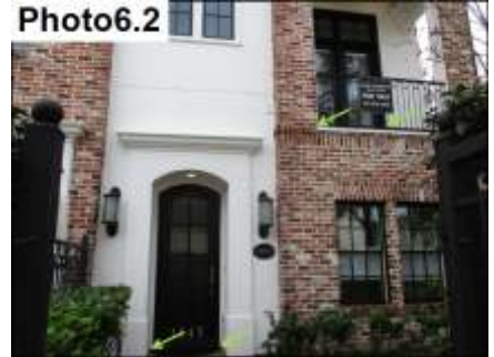
Door Trim and Miter Sealant / Maintain
