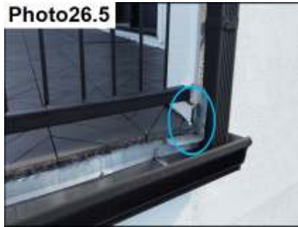
Balcony Flashing / Seal
