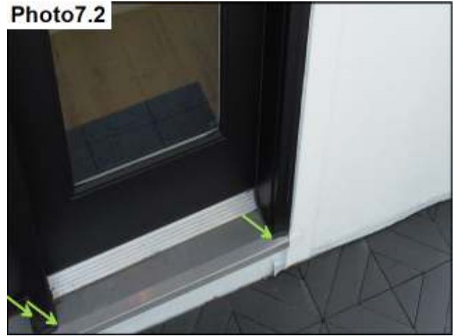
Door Trim and Miter Sealant / Maintain
