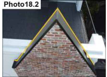
Metal Cap/Stucco Termination / Seal
