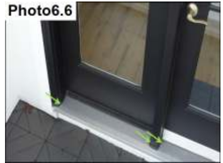
Door Trim and Miter Sealant / Maintain
