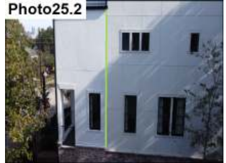
CFB/Stucco Termination / Seal
