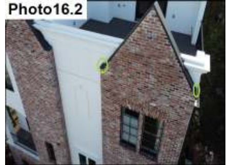
Kickout Flashing Location / Seal
