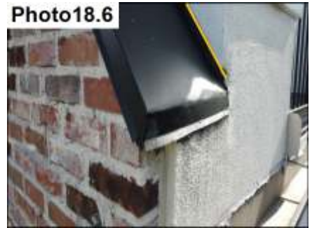
Metal Cap/Stucco Termination / Seal
