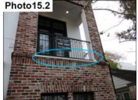
Balcony Flashing / Seal
