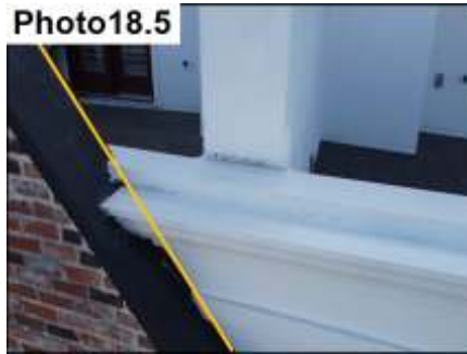
Metal Cap/Stucco Termination / Seal
