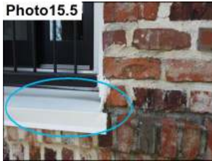
Balcony Flashing / Seal
