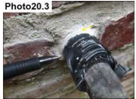
Penetration Sealants / Seal
