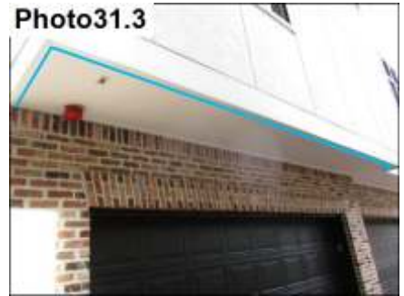
Relief Present / Clean Out Excess Sealant
