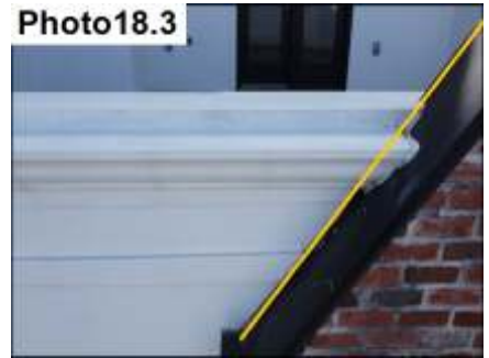
Metal Cap/Stucco Termination / Seal
