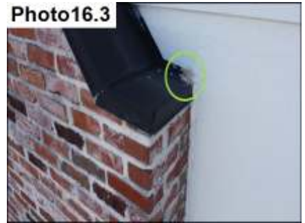
Kickout Flashing Location / Seal
