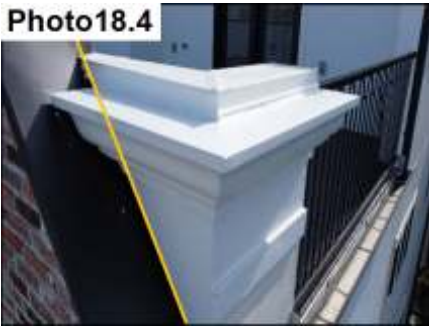
Metal Cap/Stucco Termination / Seal
