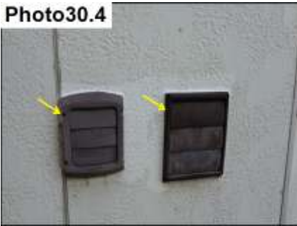
Penetration Sealants / Seal
