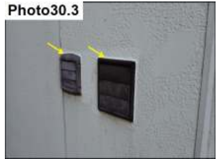
Penetration Sealants / Seal
