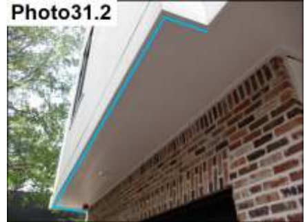
Relief Present / Clean Out Excess Sealant
