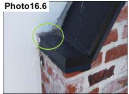
Kickout Flashing Location / Seal
