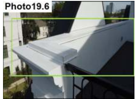
Rooftop Parapet Cap / Seal
