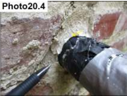
Penetration Sealants / Seal
