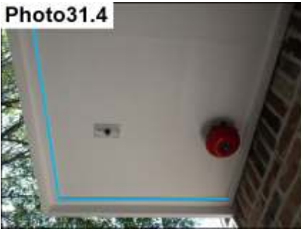
Relief Present / Clean Out Excess Sealant
