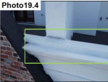
Rooftop Parapet Cap / Seal
