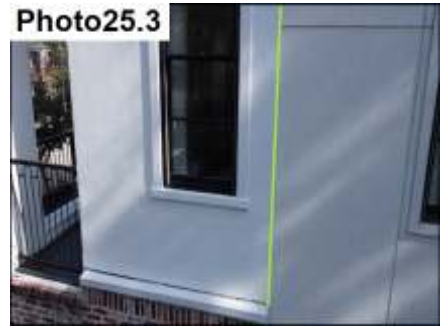
CFB/Stucco Termination / Seal
