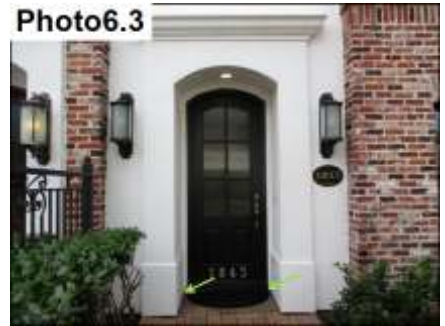
Door Trim and Miter Sealant / Maintain
