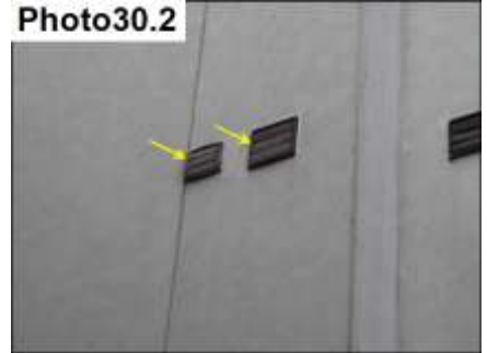
Penetration Sealants / Seal
