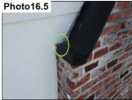
Kickout Flashing Location / Seal
