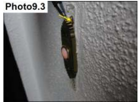
Penetration Sealants / Seal
