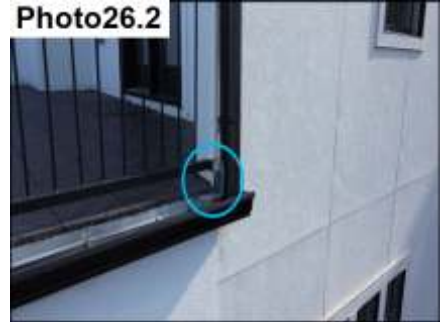
Balcony Flashing / Seal
