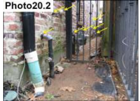
Penetration Sealants / Seal
