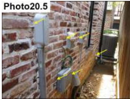
Penetration Sealants / Seal
