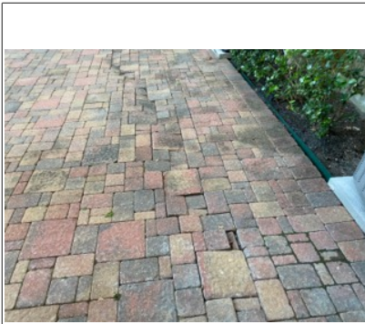
Erosion observed under pavers outside garage door.
