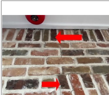
Vertical crack observed above left side of garage door. Minor settling, continue to observe the situation.
