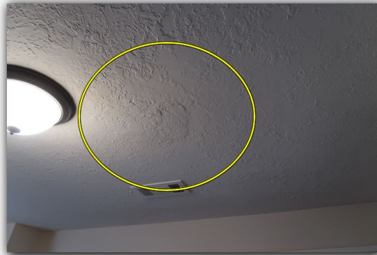
Ceiling patches, poor finish in kitchen
