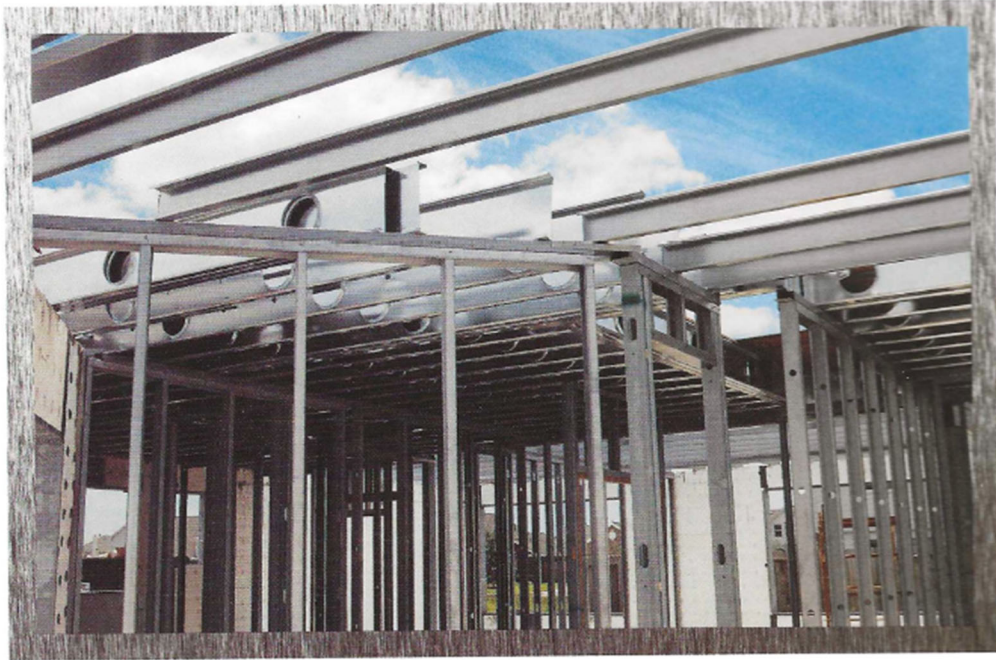
Interior wall and floor under construction using light gauge steel
