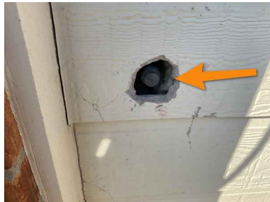
Front of the house. Right side wall. Plumbing cap.
