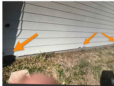
Right side of the house.
