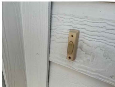
Works as intended at the time of the inspection
