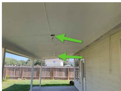
Exposed wires
