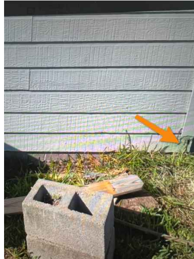
Back of the house right side corner.
