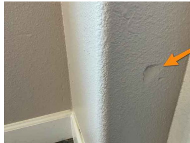
Between kitchen and living room.
