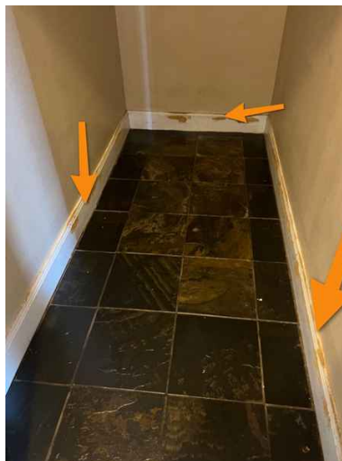
Utility room under the stairs.
