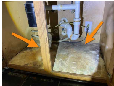
Under kitchen sink
