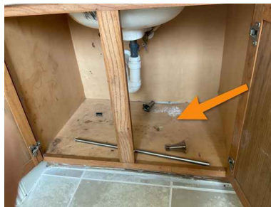
Primary bathroom under the sink.
