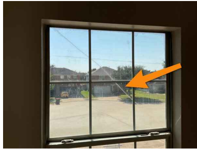
Crack window
