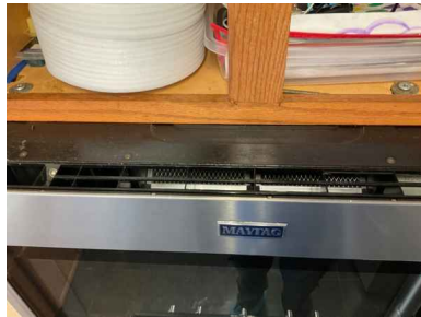
Recirculating microwave vent hood.
