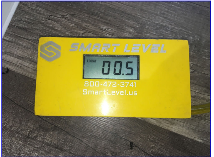
Foundation Elevation: Middle right side of home
