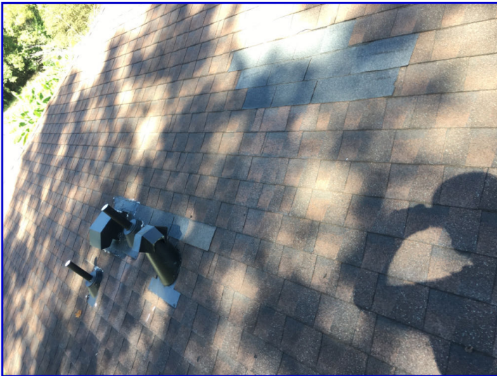
There were shingles replaced on the back side of the roof
