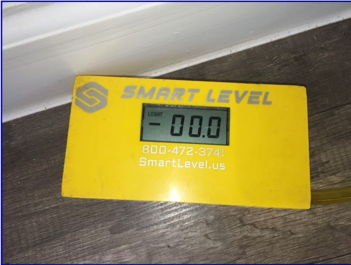
Foundation Elevation: Center of the home
