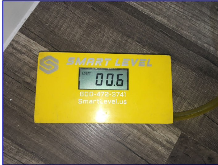
Foundation Elevation: Back right corner of home
