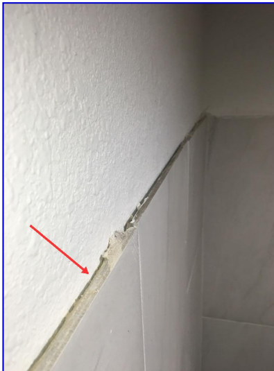
The top of the bathroom shower surround should be sealed to prevent moisture penetration
