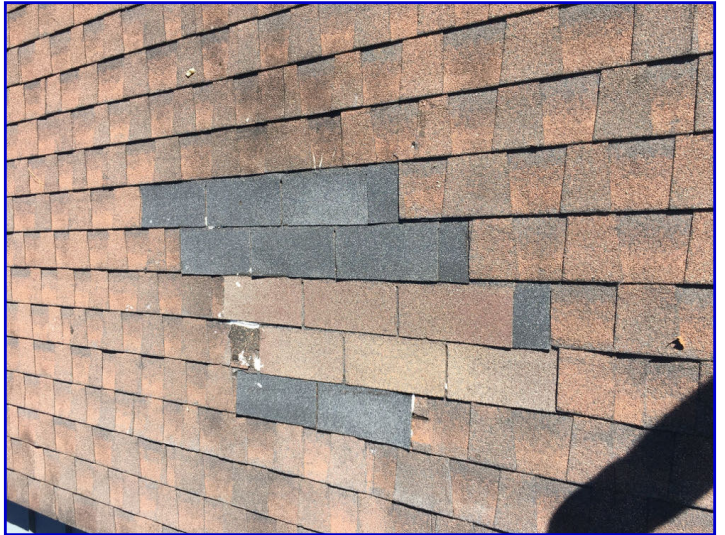
There were shingles replaced on the right side of the roof
