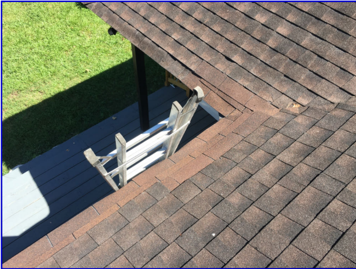
There were shingles replaced on the front side of the roof
