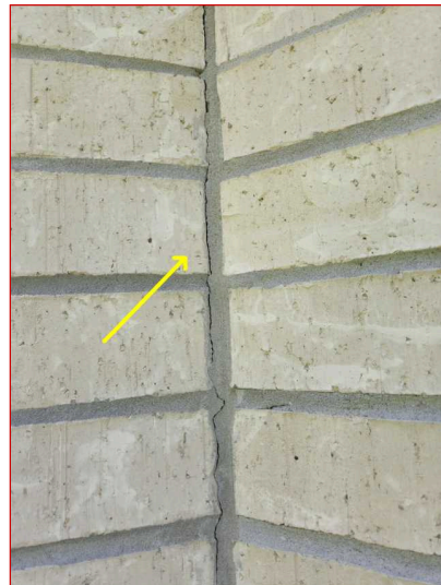
The joint tape is pulling and is sometimes related to moisture and or very minor movement of the wall(s). Sometimes this happens with homes that set without A/C for periods of time. Living room upper windows. Mortar cracks noted in one or more areas. Not uncommon to see.
