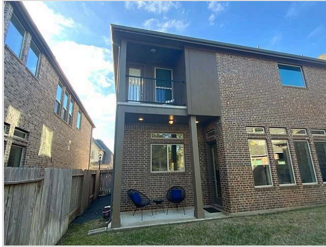
Rear porch and balcony
