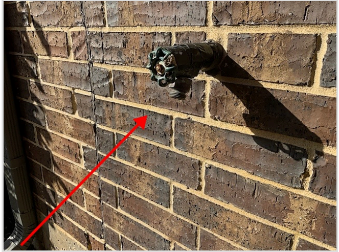
Check valves installed
