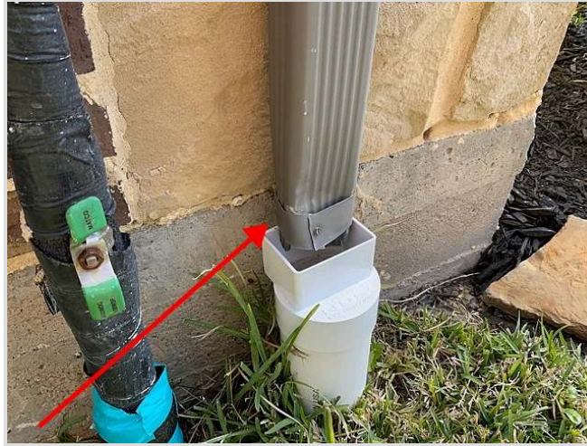
Damaged downspout
