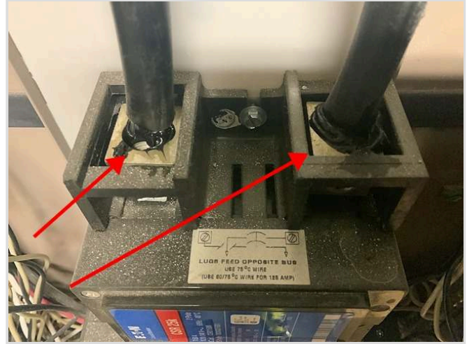
Aluminum conductors with antioxidant applied
