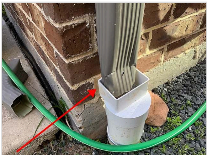
Damaged downspout
