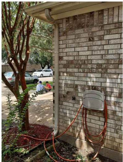
Proper grading, and drainage
