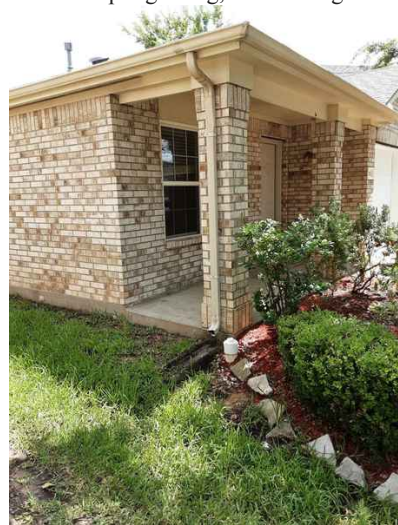
Proper grading, and drainage
