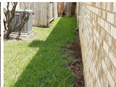
Proper grading, and drainage
