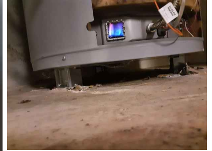
The blue flame indicates proper combustion
