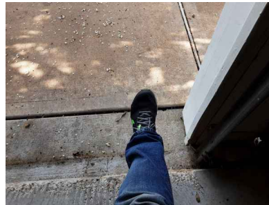
Auto-reverse sensor is operating at the time of the inspection
