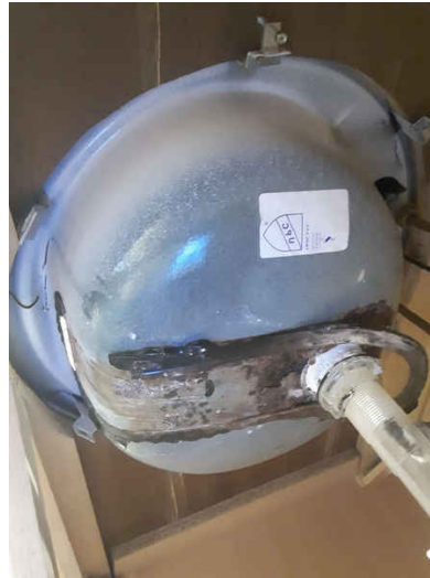
Sink overflow missing
