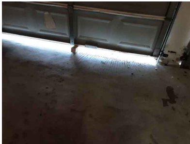
Auto-reverse mechanism is operating at the time of the inspection
