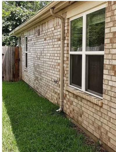
Proper grading, and drainage
