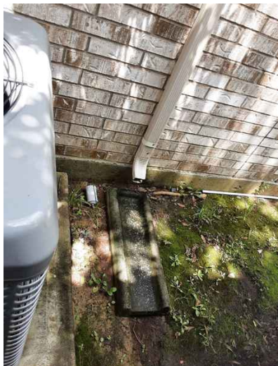
Proper grading, and drainage
