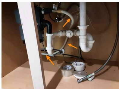
Missing Anti-syphon loop
