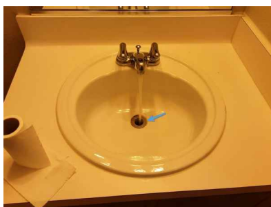
missing a stopper
