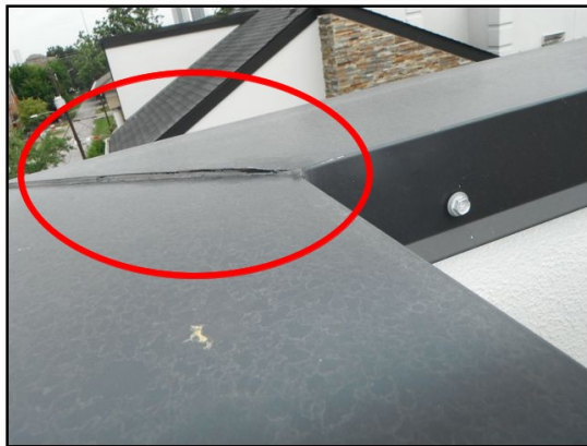
Parapet wall caps not properly sealed.
