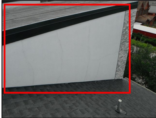
Parapet wall caps not properly sealed.
