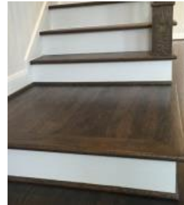
Location: Stairway Item: Stair Risers
