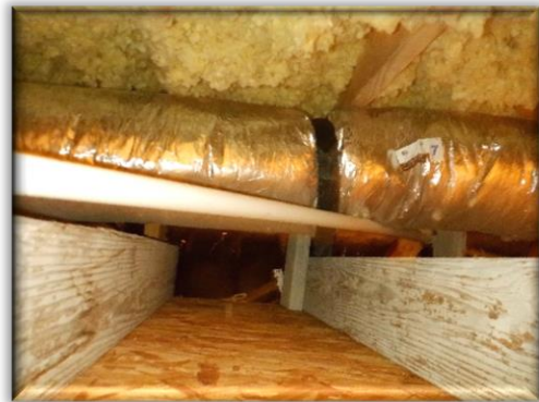
Primary drain line:
