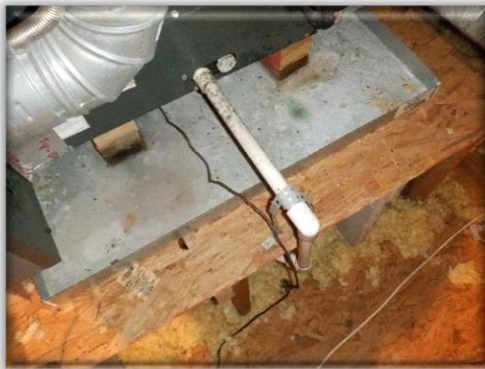
Primary drain line:
