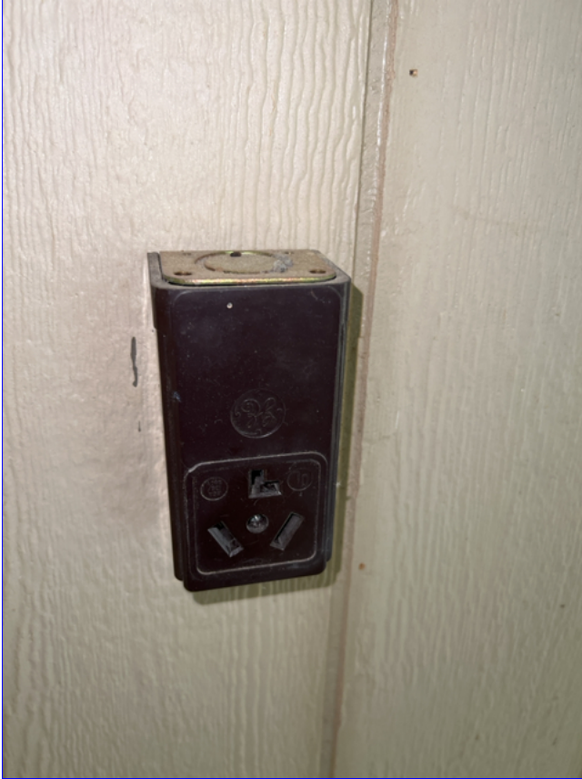
B. Photo 1(Picture) The 220 volt outlet at the dryer location, is three prong.
