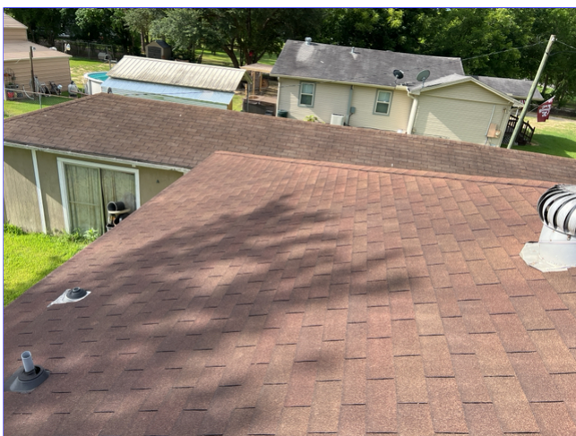
C. Photo 3(Picture) Roof pictures
