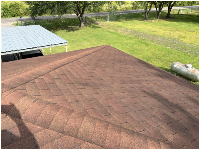
C. Photo 1(Picture) Roof pictures
