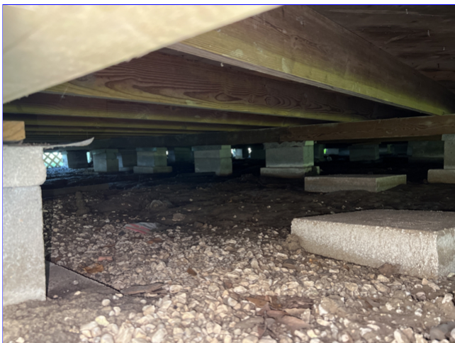
A. Photo 2(Picture) Foundation pictures.
