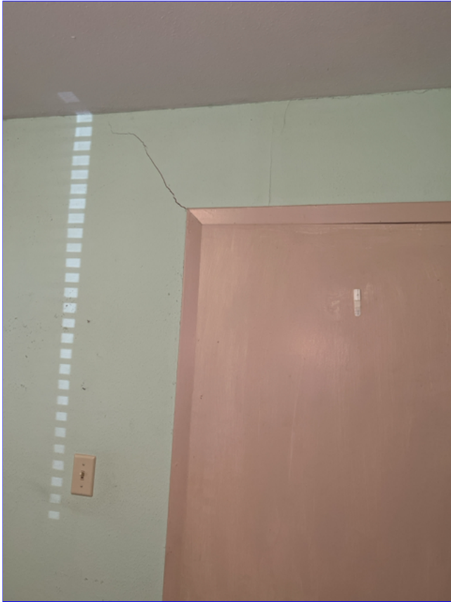
G. Photo 1(Picture) The left front bedroom door will not close because it is hitting the frame.
