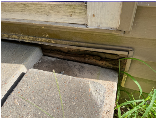
E. Photo 8(Picture) Wood rot was observed at the wall under the back door to the home.
