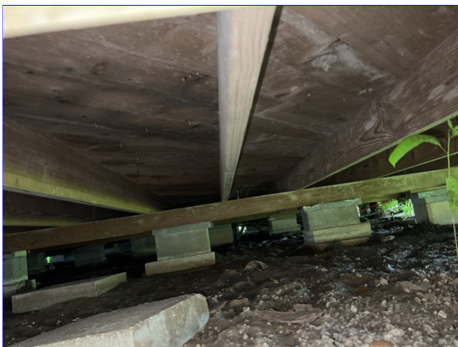
A. Photo 1(Picture) Foundation pictures.
