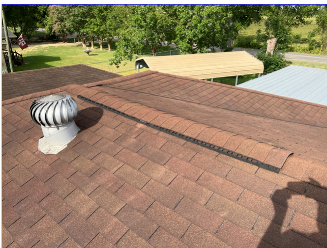
C. Photo 2(Picture) Roof pictures
