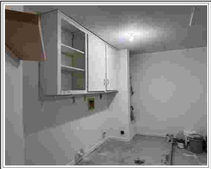
LAUNDRY AREA IN GARAGE
